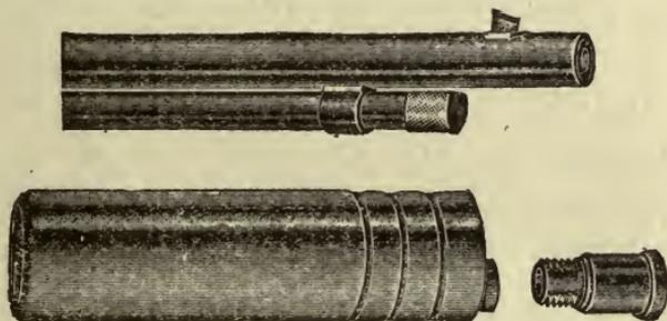
Through the silencer, lengthwise, there is a clear passage for the bullet and surrounding the passage are laminae for whirling and retarding the powder gas. In its present form it is a sort of necessary evil: a crude protuberance performing an incomplete function. The interested rifleman may yet simplify and improve it, thereby conferring a benefit and receiving, perhaps, a fortune.
