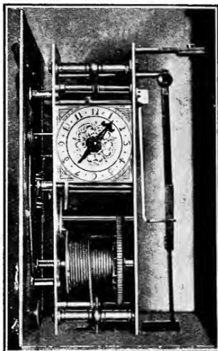
FIG. 656.—Side view of Time-piece Movement, by William Clement, about 1676.
