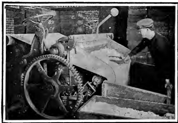
FIG. 278.—Running Pulped Nitrocellulose through the "Wet Machine."
