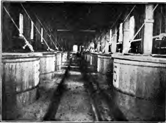
FIG. 287.—Nitrocellulose Wash House.
