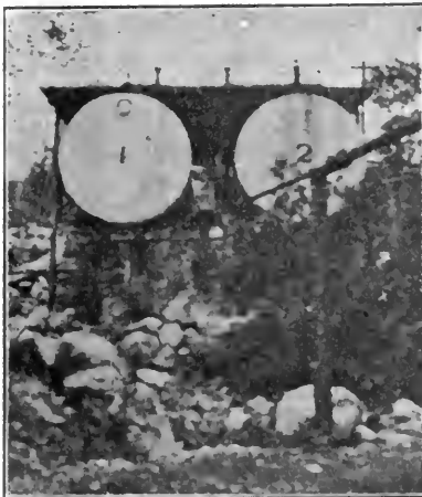
FIG. 25.—Nitrating Acid Storage Tanks.
