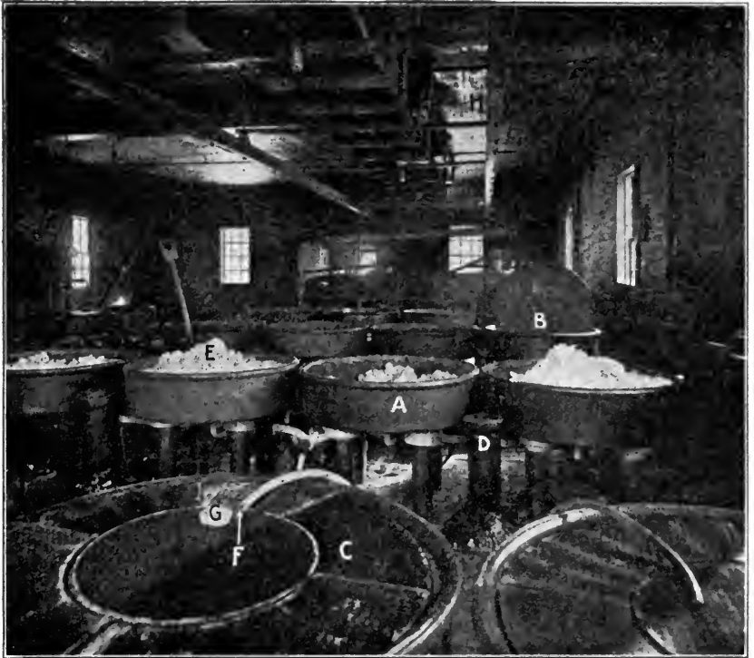
FIG. 12.—The Thomson Displacement Process for Cotton Nitration, at Picatinny Arsenal, Dover, N. J.
