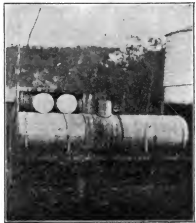
FIG. 26.—Nitrating Acid Storage Tanks.
