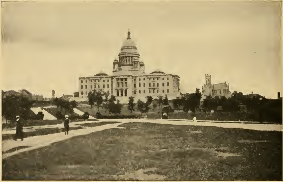
The Rhode Island State House at Providence
