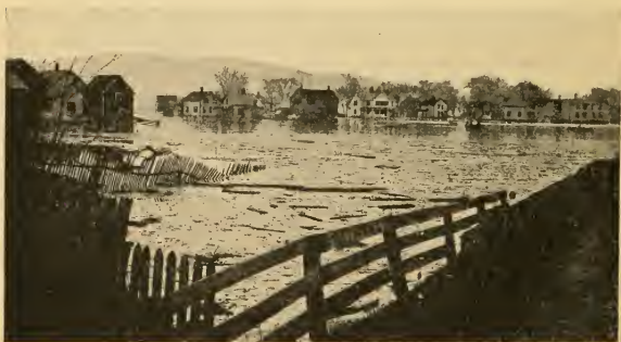
High water on the outskirts of Northampton
