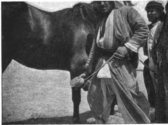
Showing the solid steel shoe with small hole in center.
