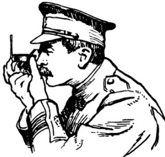
FIG. 21.—THE USE OF THE PRISMATIC COMPASS (OLD PATTERN)
