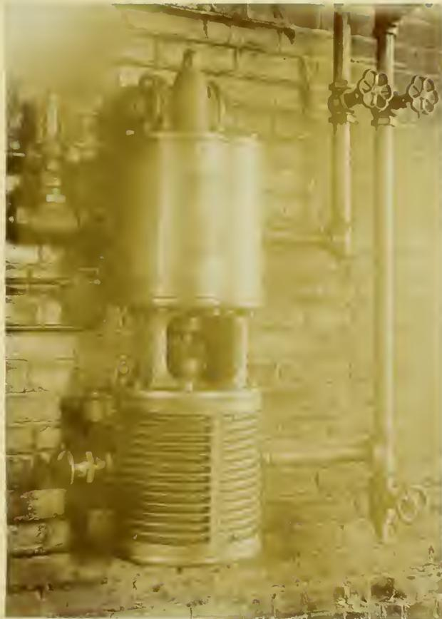
During the test run on the Downie pump the water was pumped into a tank of known area. The height of water at beginning of test was carefully noted and also at the end of test. It was thus possible to obtain the number of cubic feet of water pumped into the tank.
