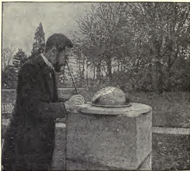
FIG. 56.—BESSON'S SPHERICAL MIRROR NEPHOMETER.
