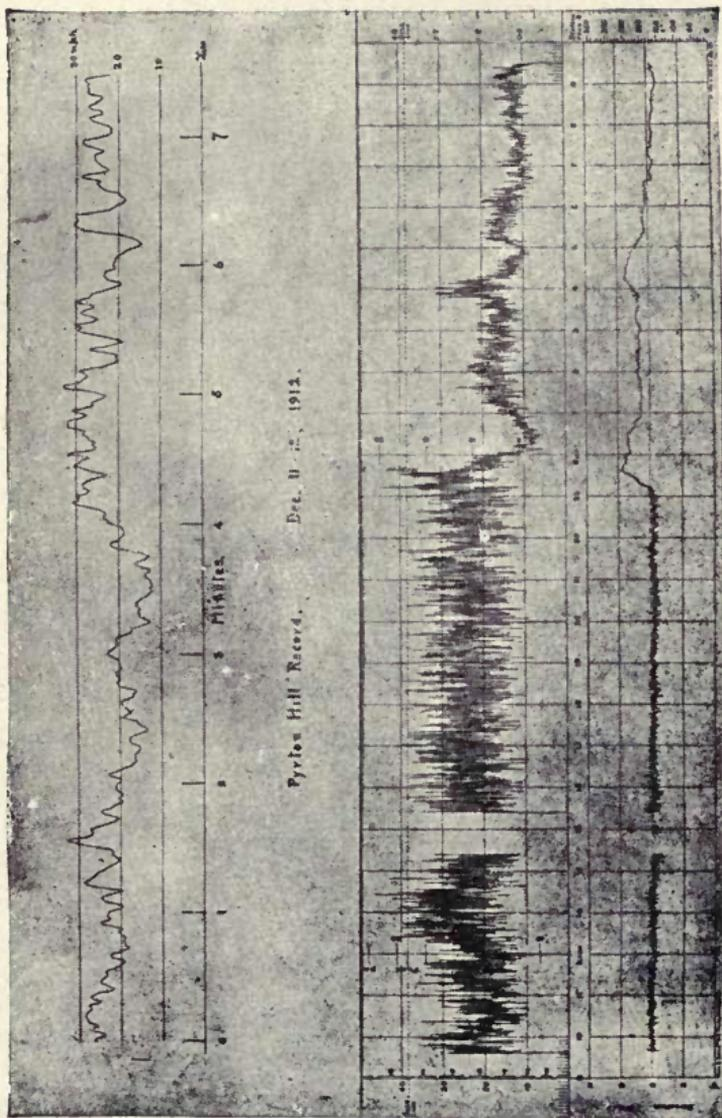
FIG. 12—WIND RECORD BY PRESSURE-TUBE ANEMOMETER,
