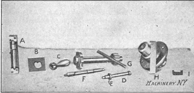
Fig. 15. Gages for Testing the Parts of the Device shown in Fig. 13
