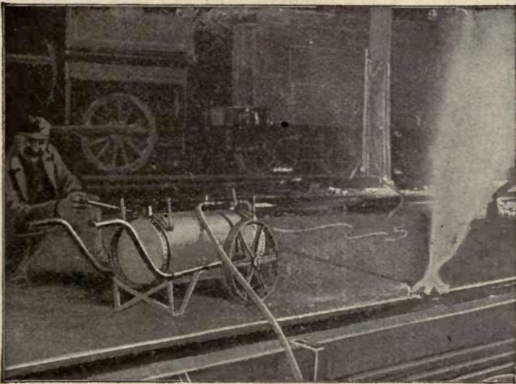
portions of oil and air. The tank is most conveniently mounted on a truck, by which means it may be easily removed from one part of the roundhouse to another.
