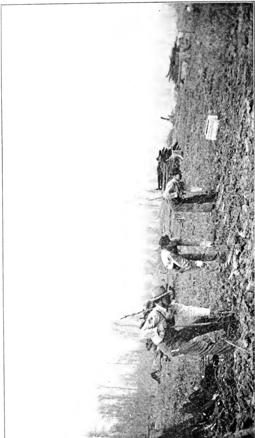
PUNCHING THE HOLES FOR DITCH BLASTING
