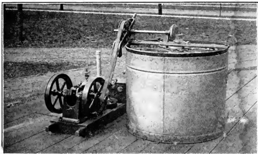
AN EIGHT-FRAME EXTRACTOR CONNECTED TO A ONE HORSE
