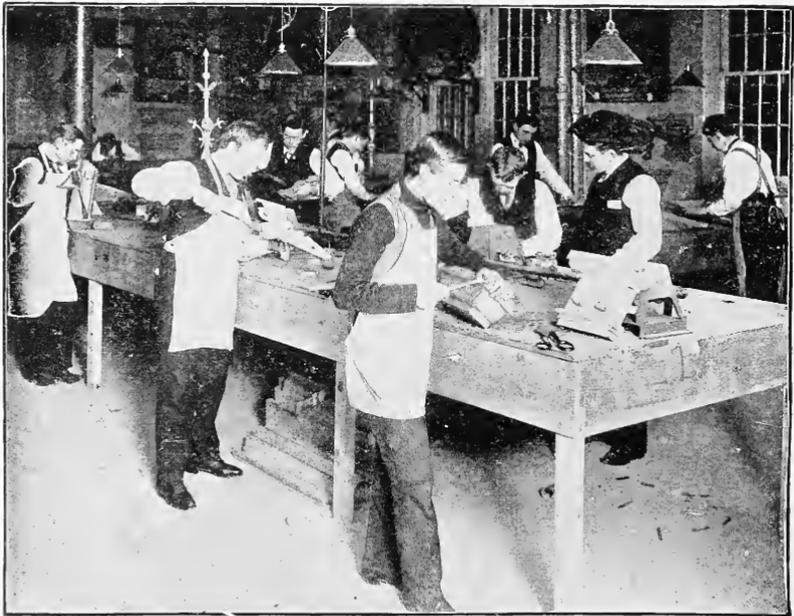
FIG. 81. Trade School Students at Work Joining Molded Gutter.
