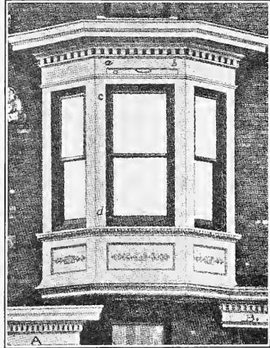
FIG. 516. Leveling Bay Window in Attaching to Building.
