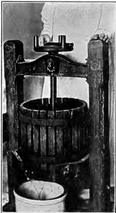
FIG. 21. Pressing Crushed Fruit.
