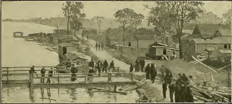
Fig. 100. — A Mississippi levee, Greenville. High water above the level of the town.
