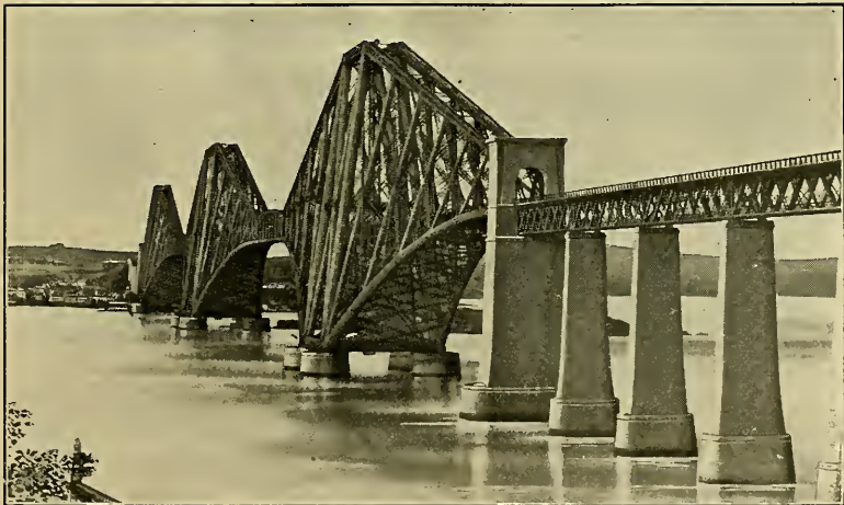
Fig. 297. — Forth bridge, Scotland.
