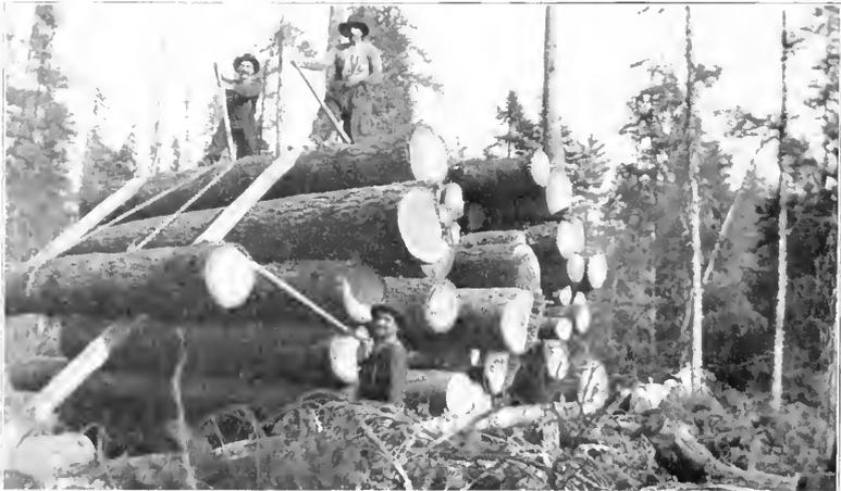
Fig. 11. Decking Logs on Skidway.
