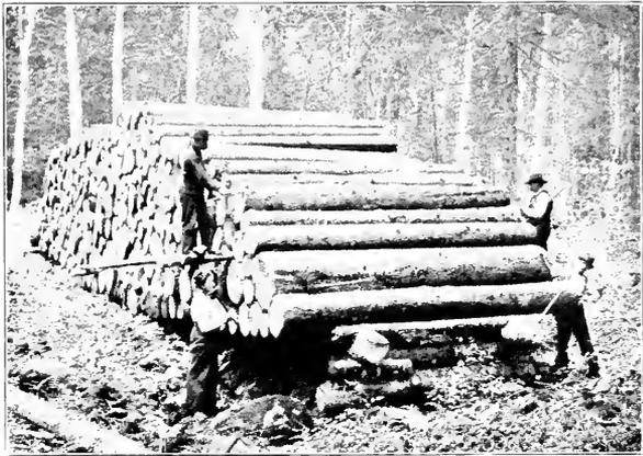
Fig. 9. "Scaling" Logs on the Skids.
