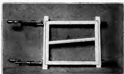
Fig. 253. Gluing Together a Picture-Frame (See also Fig. 254.)
