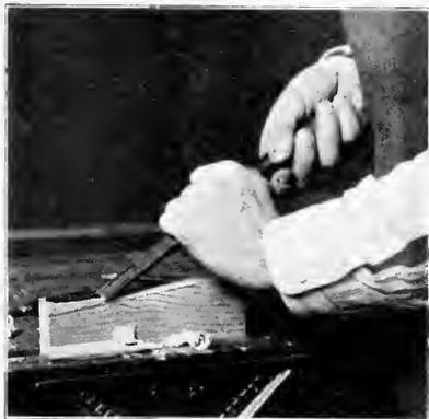
Fig. 69. Paring With a Chisel.
