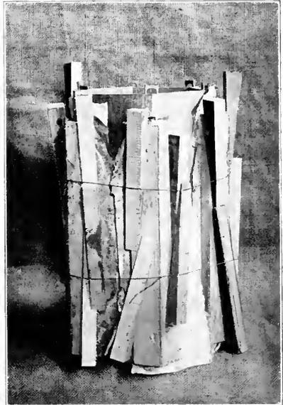
Fig. 256. Gluing up a Column Joint.
