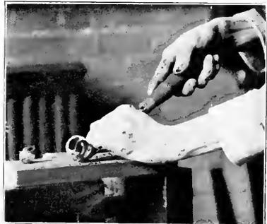
Fig. 82. Gouging.
