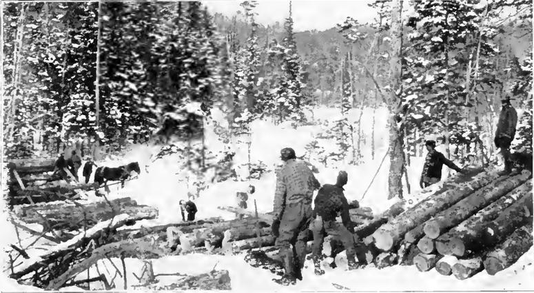
Fig. 12. Loading a Sled from a Skidway.
