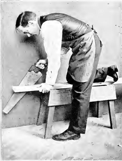
Fig. 88. Rip-Sawing on a Horse.
