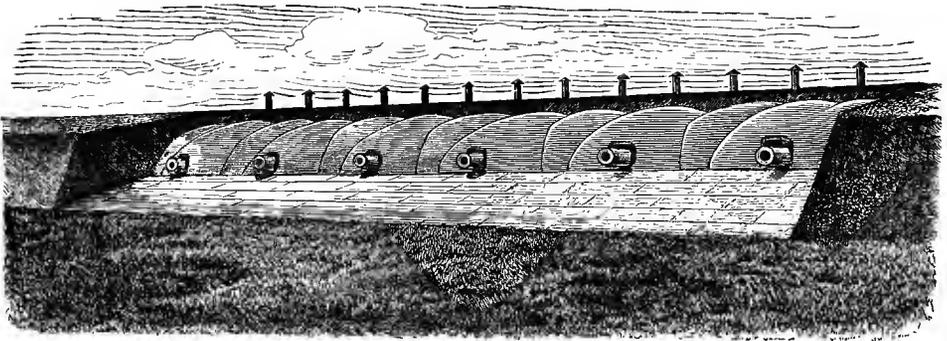
The adjoining edges of the several plates are planed to a flat surface, and each edge is provided with a groove, into which zinc is cast when the battery is mounted, or iron keys inserted. Owing to the weight of the plates no further fitting is necessary.
