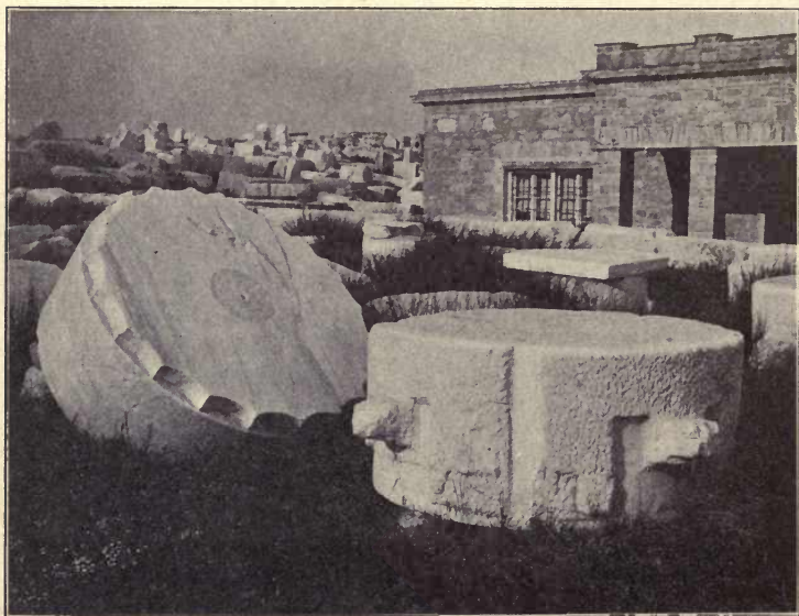
FIG. 9. — Tenons for lifting drums of columns.
