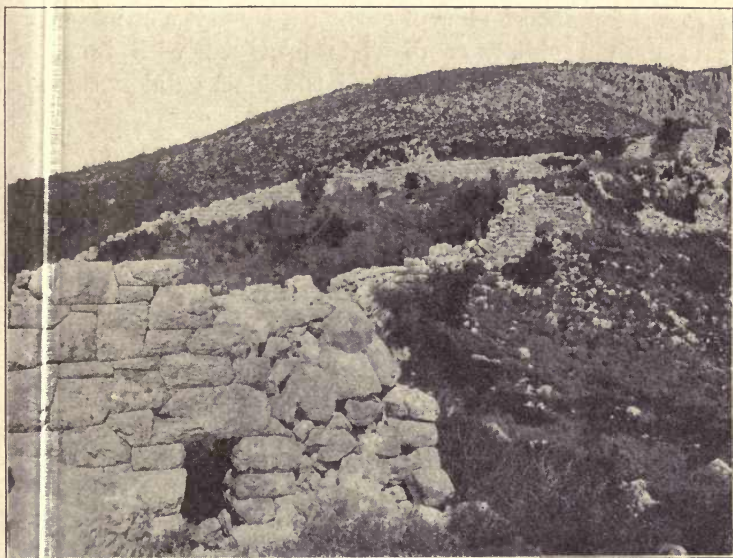
FIG. 12.—Polygonal masonry from Samikon.
