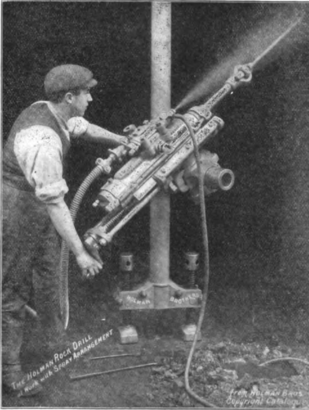
THE "HOLMAN" ROCK DRILL WITH PATENT SPRAY.
