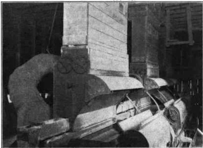
FIGURE 19.—Small-drum cleaning feeders, with pneumatic distribution system.
