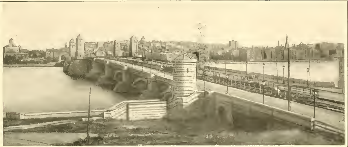
Cambridge Bridge across the Charles River to Boston
