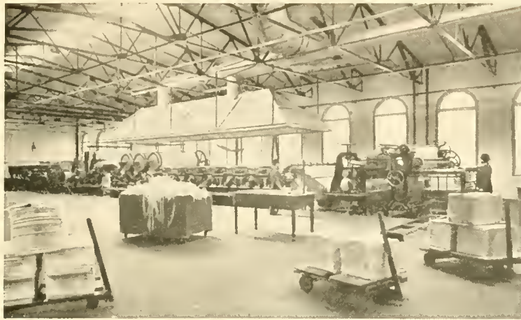
Machine room in a paper mill, Holyoke
