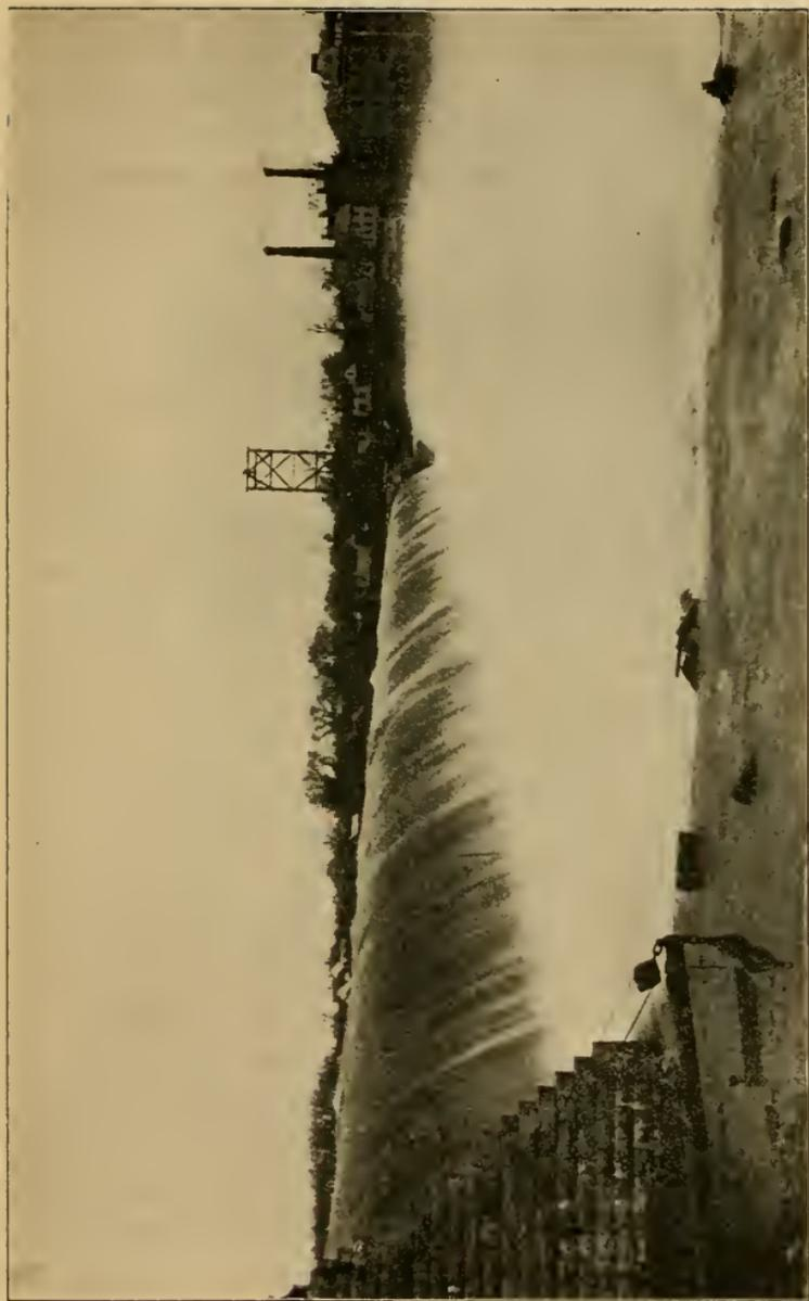
FIG. 8. The Great Dam at Holyoke ; 35 Feet High, about 1000 Feet Long, and with 12 Feet of Water on the Crest.
