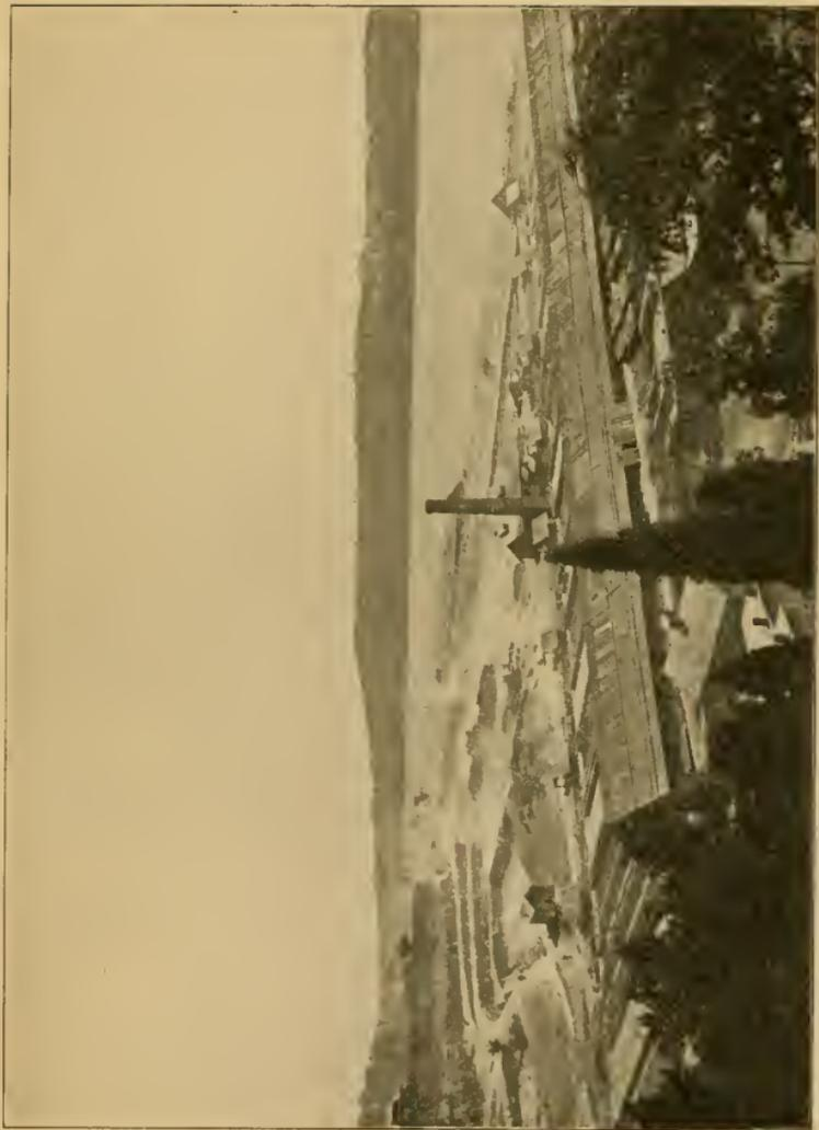
FIG. 5. Roseton Clay Beds and Brickyards, on the Hudson. The Terraces are due to the cutting of the Clay to Successive Levels. Photograph by H. Ries, in "Bulletin of New York State Museum."
