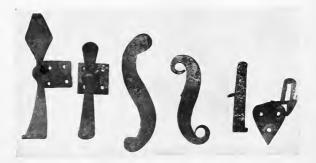
A SERIES of Shutter Fasteners. The modern blind was first used in the last decade of the 18th Century, in one large old coast town. The spring fastener on the right was the latest and poorest type. It continually got out of order. The others are earlier, operate by gravity and cannot go wrong. The crude S fasteners should be compared with the somewhat later design, 390 on the next page. The types at the left are later than the S type, since they are attached by plates.
