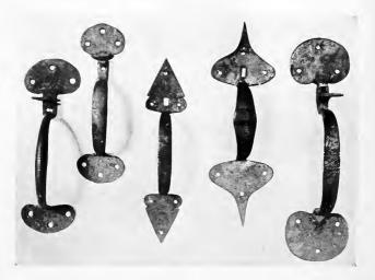
THE Fourth Latch in the line above is found on many good houses. It is the best design of the five. The handle portion is shaped more than in the others. This one was on the back door of the Wentworth-Gardner house. It was used as an inside and outside latch, in differing sizes.
