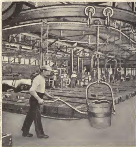
Fig. 140. Overhead Track and Trolley.
