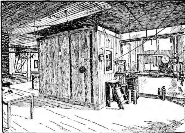
ATWATER'S RESPIRATION CALORIMETER.
