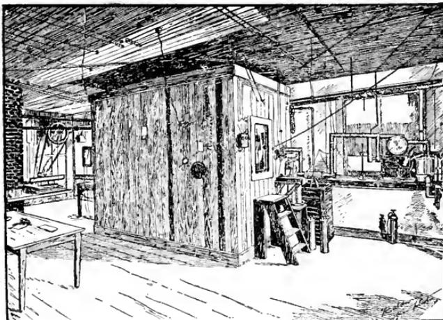
ATWATER'S RESPIRATION CALORIMETER.
