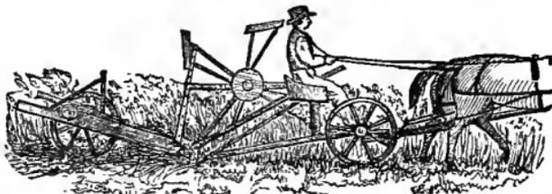
*Manny's Mowing and Reaping Machine, showing the reel distinctly.*
