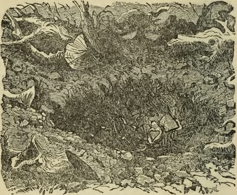
Fig. 44.—THE EFFECT OF BLASTING THE STUMP.
