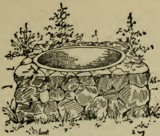
Fig. 221.—A SPRING WALLED UP.
