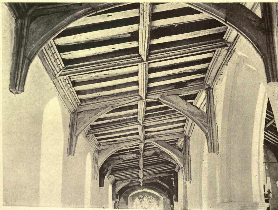
SOUTHACRE, NORFOLK, FLYING BUTTRESS ROOF OF AISLE
