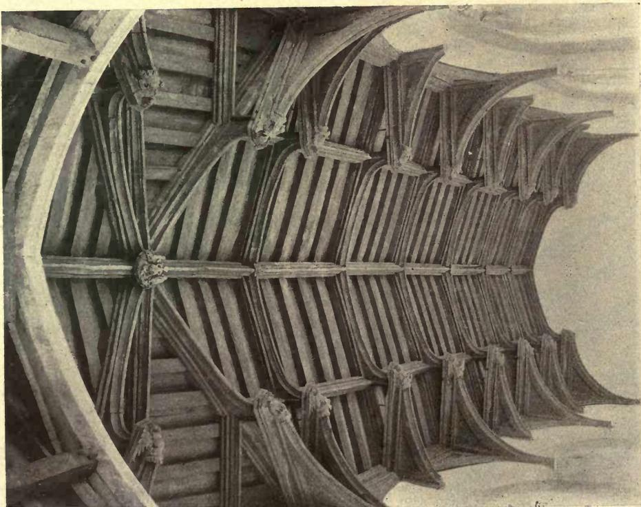
THE TRUE DOUBLE HAMMER-BEAM ROOF
