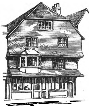
FIG. 176. WEATHER-TILING, HOUSE IN SALISBURY
