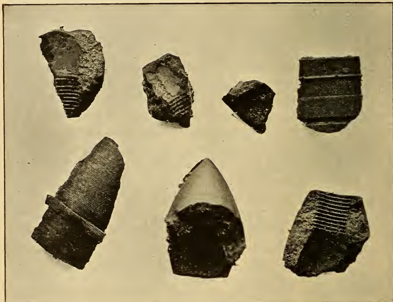
FIG. 93.—Fragments of Vickers-Maxim one-pound shell. (Makins.)
