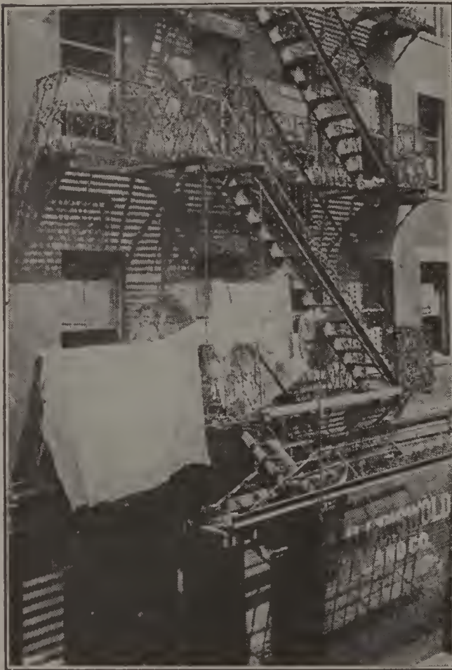
HOW NOT TO USE A FIRE ESCAPE.
