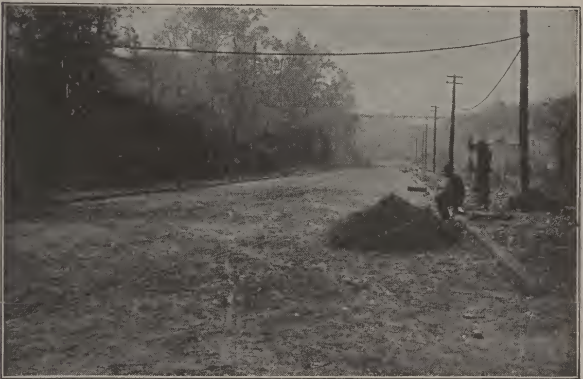
GRADING OF A STREET COMPLETED.
