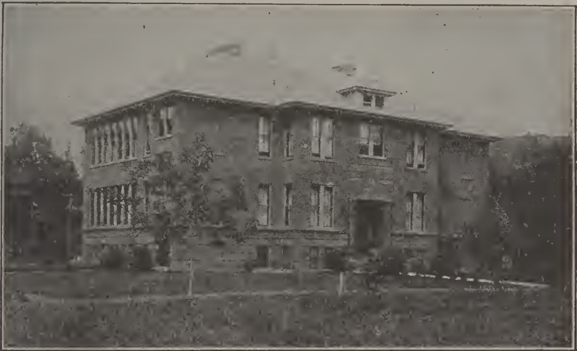
AN EXCELLENT SCHOOL BUILDING IN A COUNTRY VILLAGE.
