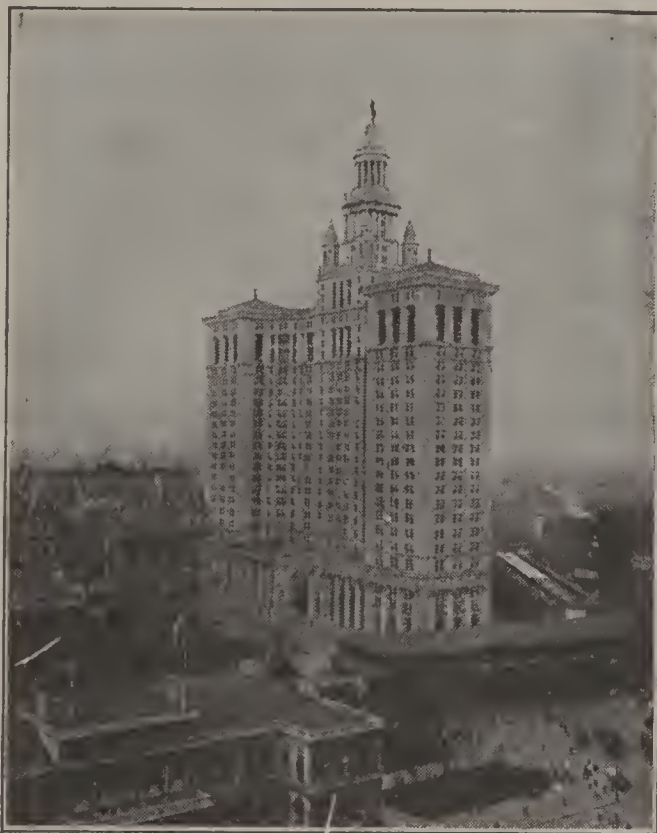
THE MUNICIPAL BUILDING, NEW YORK CITY.
