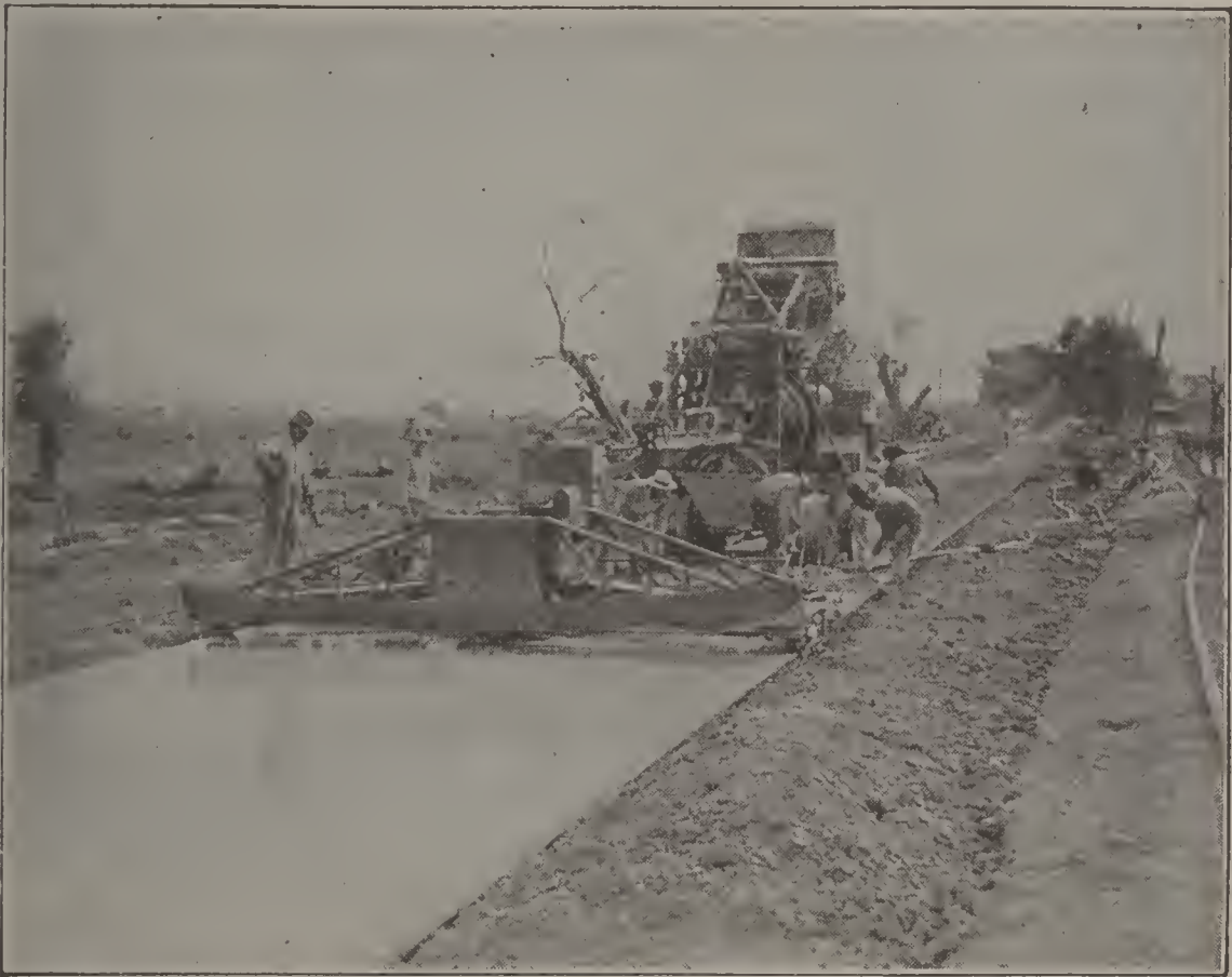
Courtesy Portland Cement Association CONSTRUCTING A CONCRETE ROAD.
