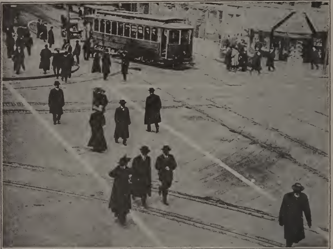
SAFETY LANES FOR PEDESTRIANS.
