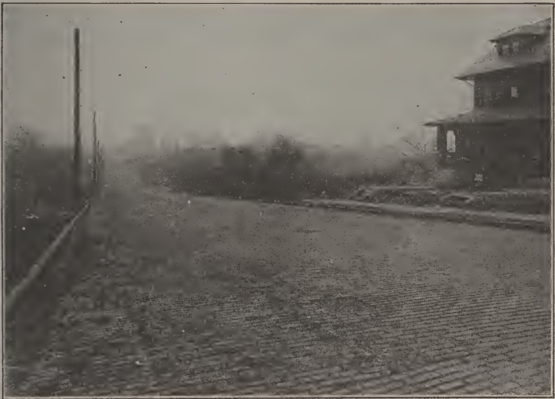
BRICK PAVEMENT ON A CITY STREET.
