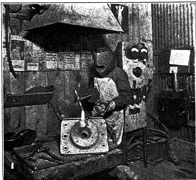
FIG. 13.—Carbon-Arc Welding, Using King Mask.
