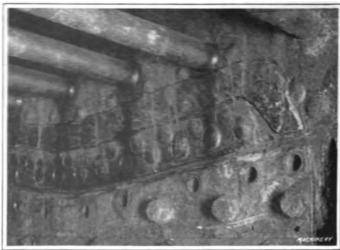
Fig. 35. Patch shown in Fig. 34 after being welded in Place
