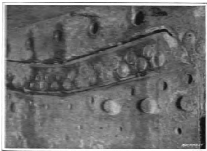
Fig. 34. Patch riveted to Metal-ting Ready for Welding
