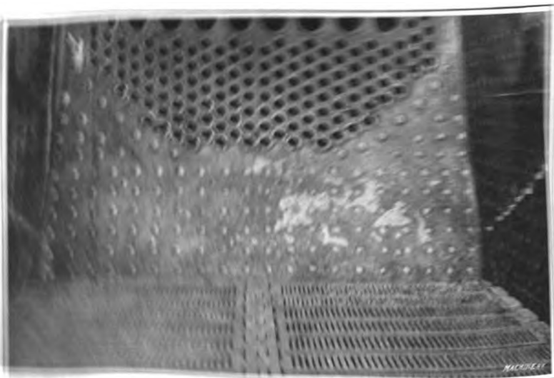
Fig. 1. Boiler with Electrically Arc-welded Flue Sheets, Tubes, and Heater Tubes, and Brick Arc Studs
