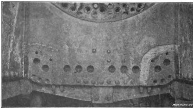
Fig. 17. Completed Weld with Sections of the Throat Sheet replaced
