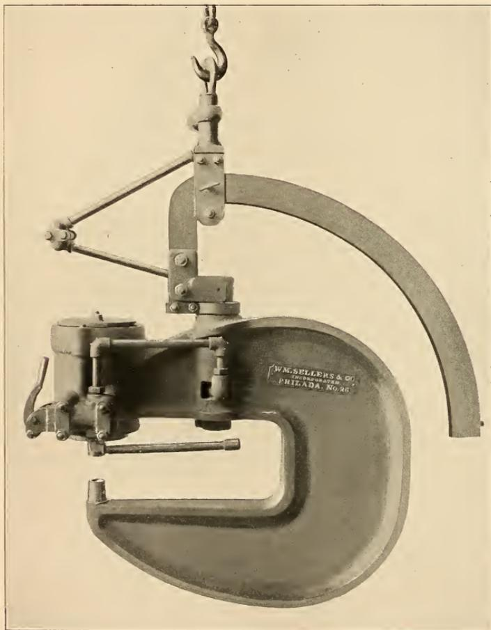
DIRECT-ACTING PORTABLE HYDRAULIC RIVETER.
