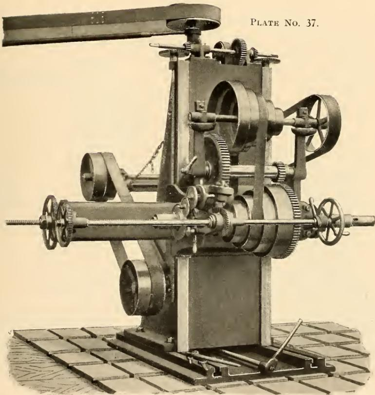
FLOOR-BORING MACHINE—DRIVEN BY BELT AND SWING FRAME.
