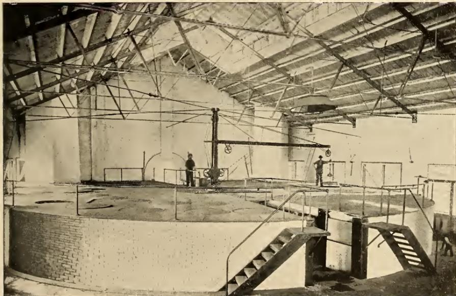
HYDRAULIC CRANE.—FOR THE ANNEALING FURNACE OF THE WHEEL
