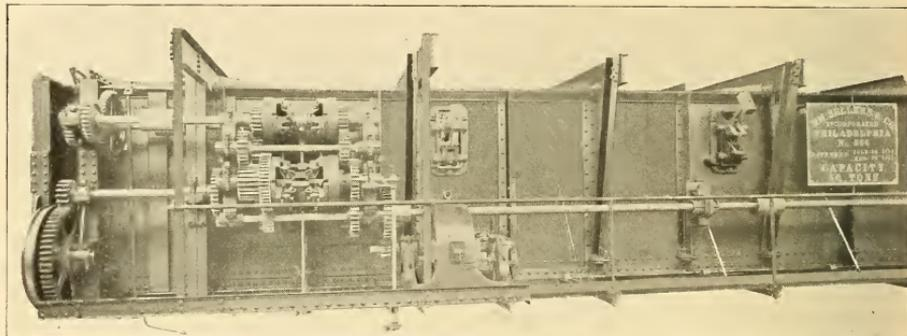
50-TON TRAVELLING CRANE.—SINGLE MOTOR TYPE.
