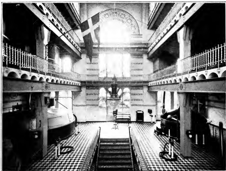
Interior from Ny Carlsberg Brewhouse, Copenhagen.
