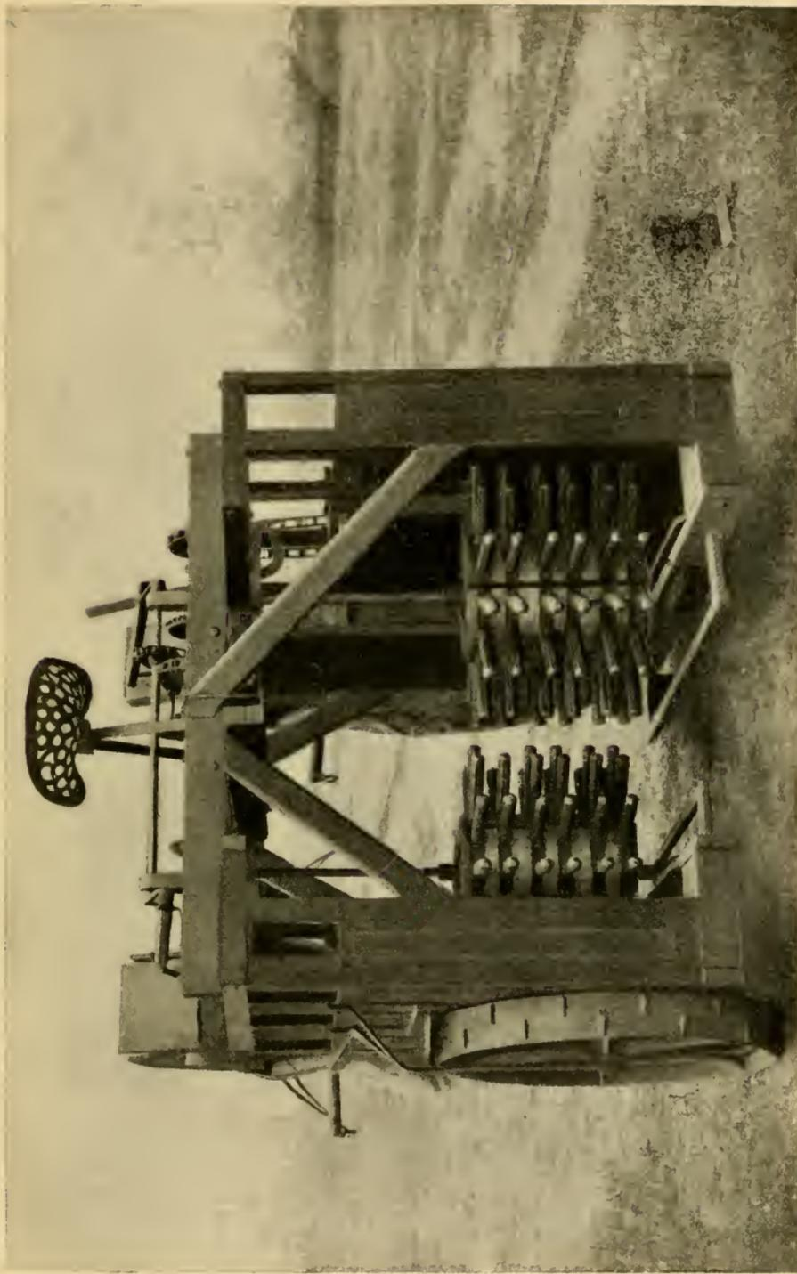
FIG. 56. Experimental Cotton Picking Machine; Rear View
