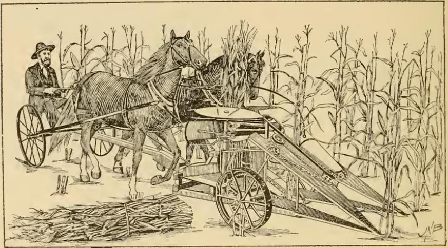
FIG. 11.—Vertical corn harvester in the field.
