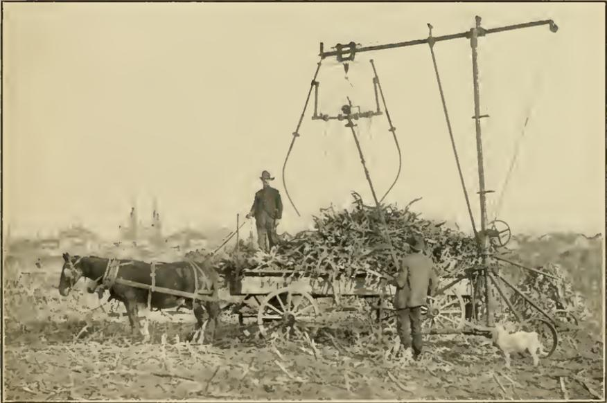
FIG. 2.—CORN-SHOCK LOADER, EMPTY.
