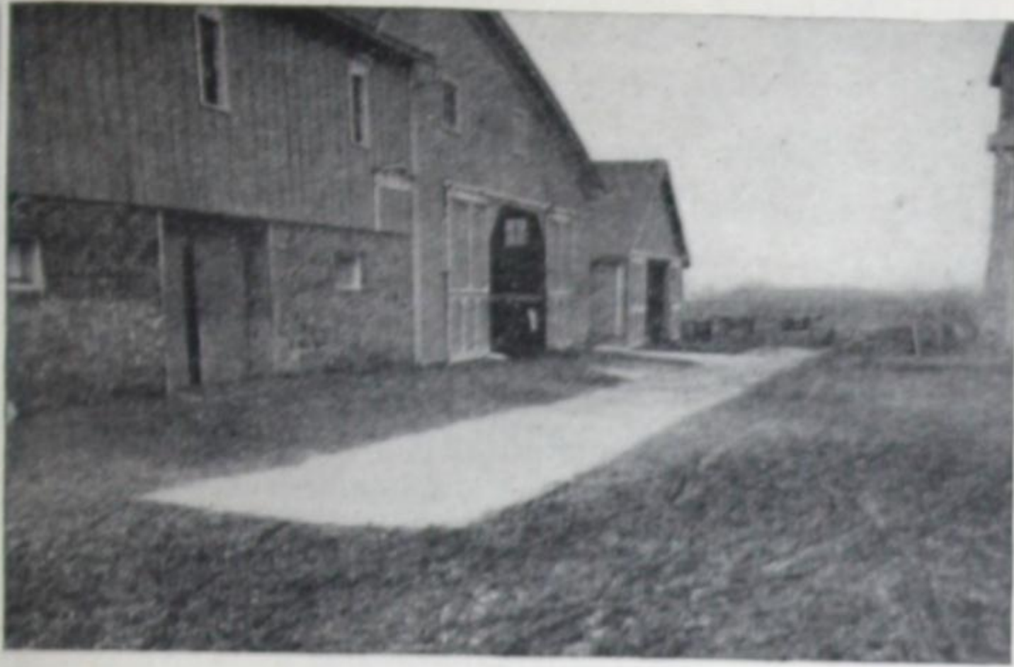
Fig. 49—Concrete driveway around barn. The rutted dirt at the side shows how much harder hauling is without the concrete driveway.
