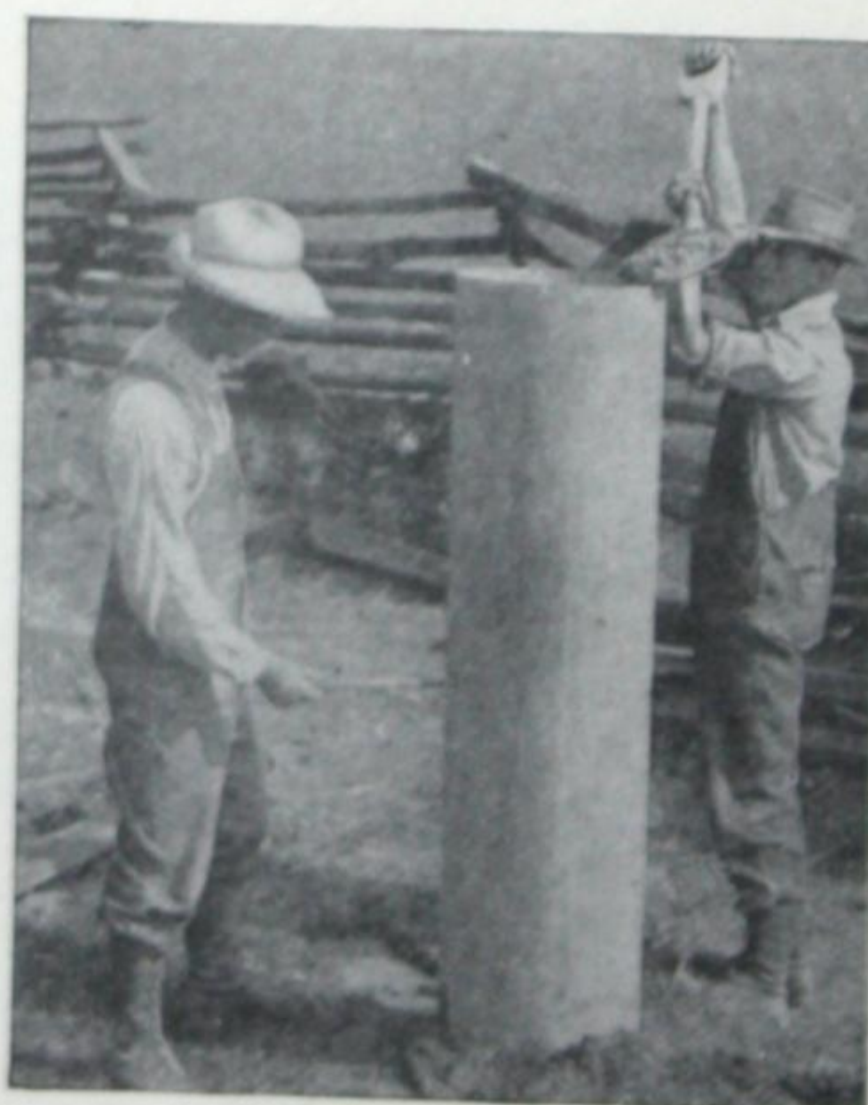
Fig. 145—Working on a concrete corner post. Filling the form and steadying the reinforcing rods.
