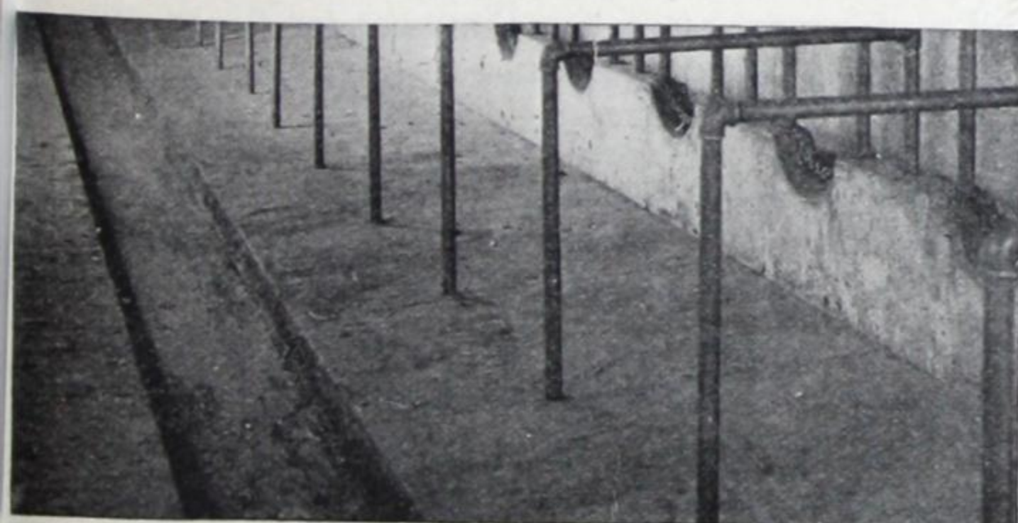
Fig. 65—Cow barn with concrete manger, stall floor, gutter. The concrete gutter saves liquid manure, and helps keep the cows clean and healthy.
