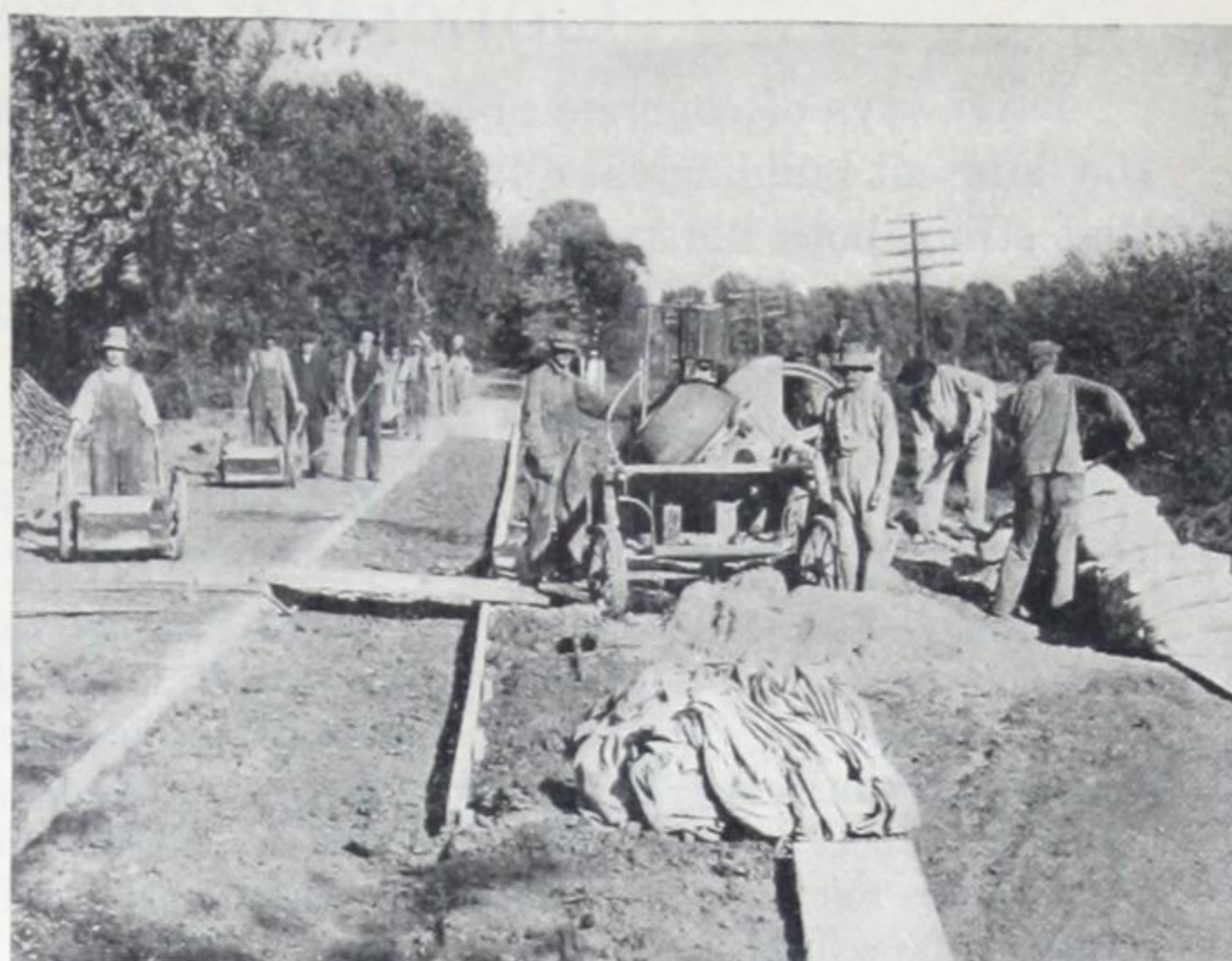
Fig. 46—A large paving job, with machine mixer.
