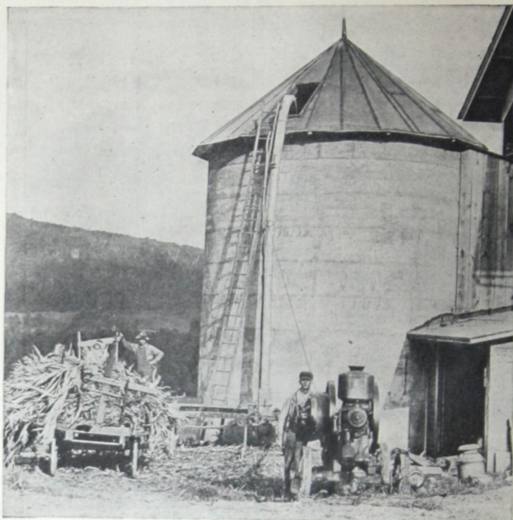
Fig. 107—Filling a concrete silo with corn stalks.
