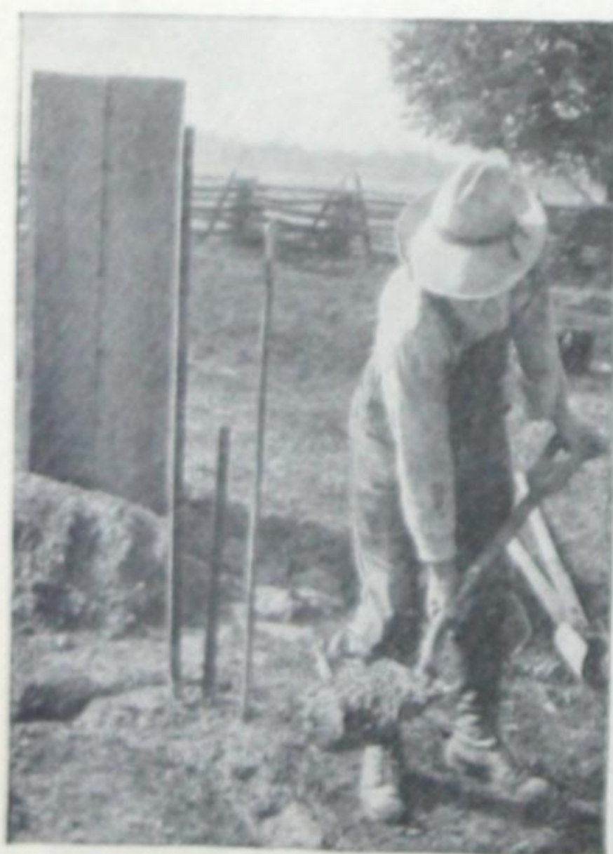
Fig. 144—Working on a concrete corner post. The reinforcing rods are embedded in the foundation.
