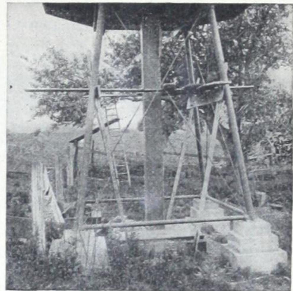
Fig. 31—Piers for a water tank foundation.
