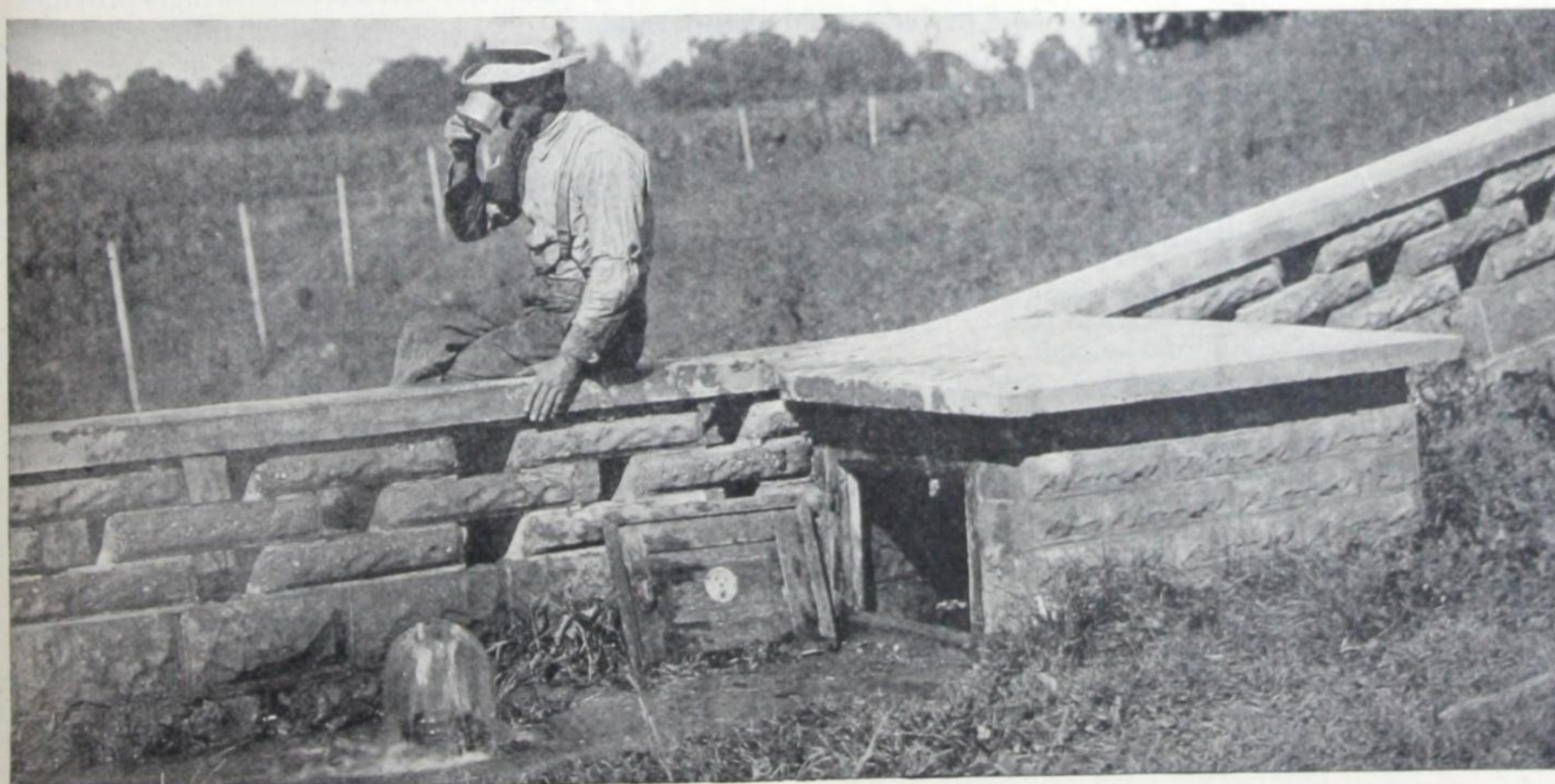
Fig. 85—Concrete block box for hydraulic ram with wall built of spaced concrete blocks on heavy block foundation.
