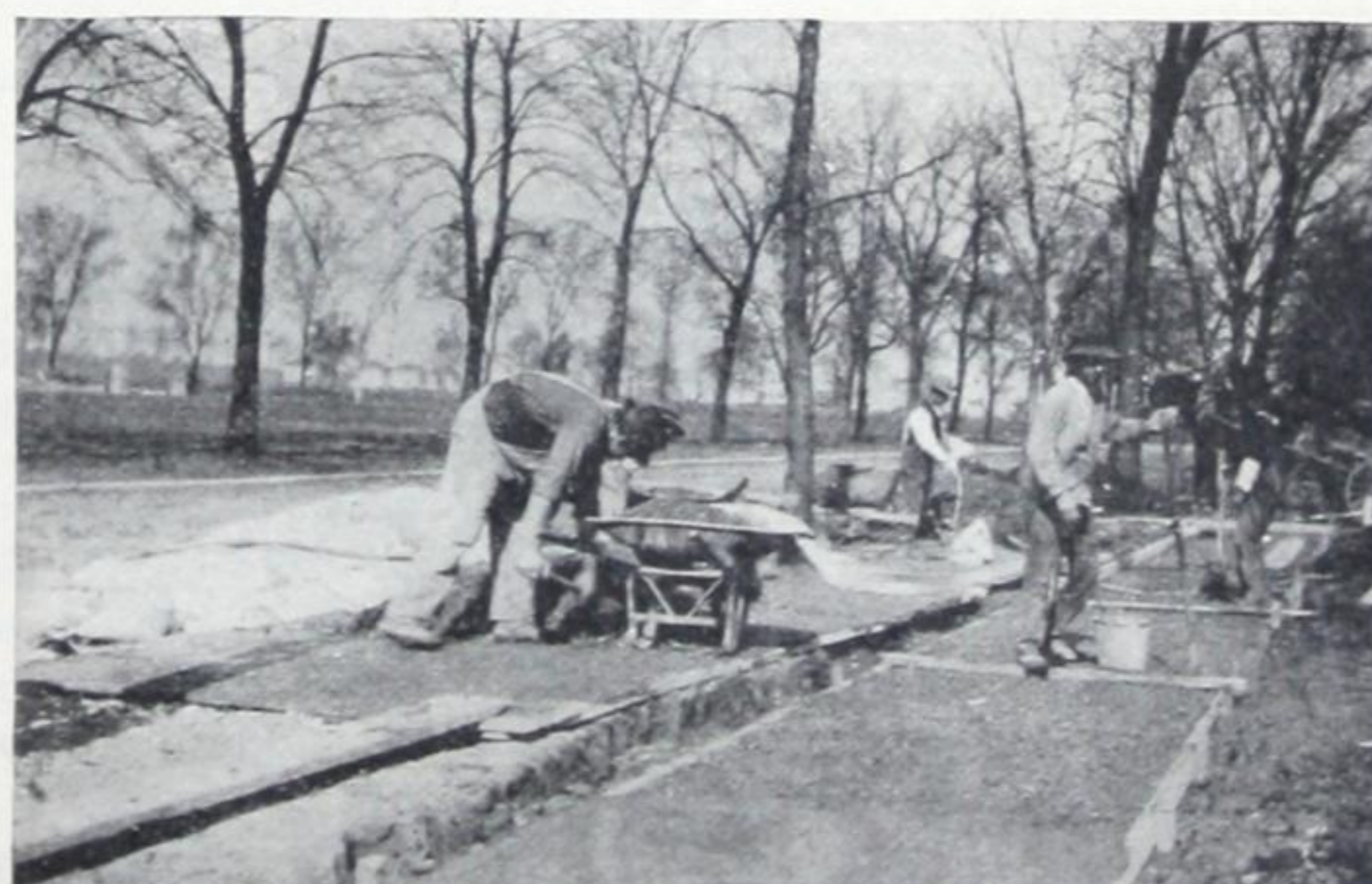
Fig. 48B—A small paving job. Four men at work—one mixing by hand, one carrying with wheelbarrow, one filling the forms, and one tamping.
