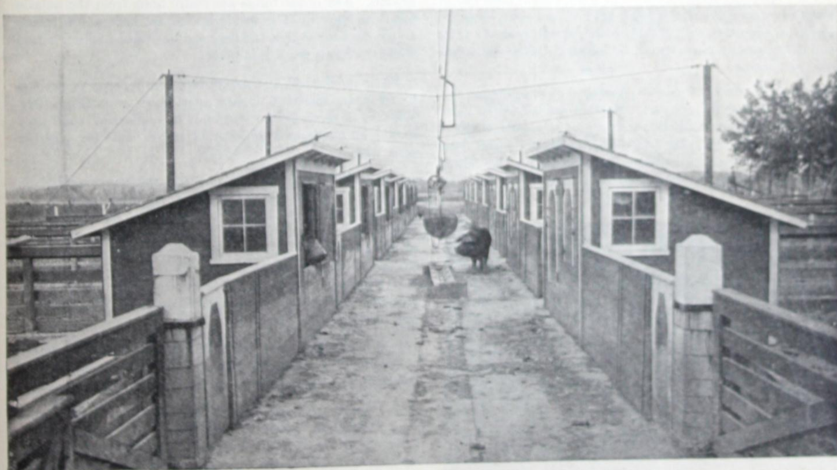
Fig. 112—Concrete aisle between two rows of hog houses with feeding troughs.
