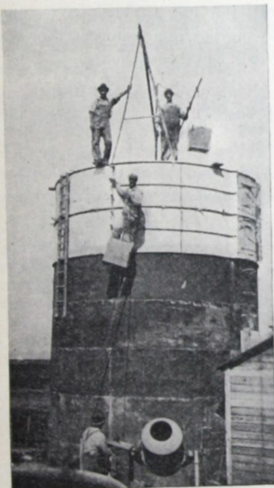
Fig. 105—Showing small machine mixer, block and tackle and forms for building silo or large tank.
