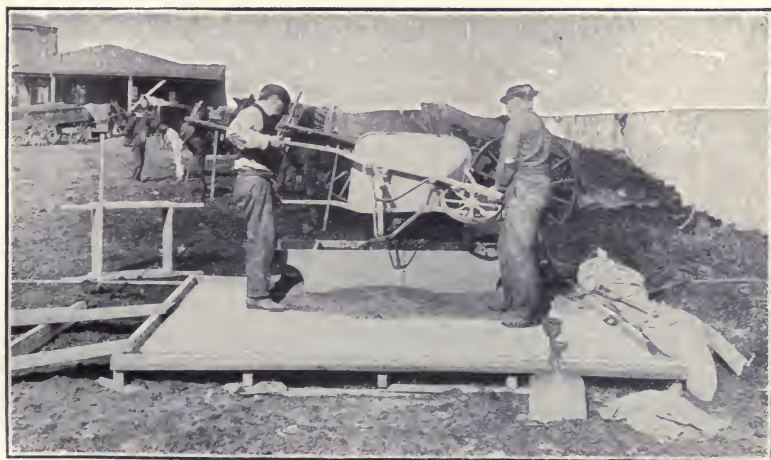
Fig. 7.—Filling the Stone (or Gravel) Measuring Box—First Method.
