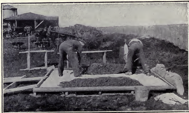
Fig. 10.—Mixing the Stone (or Gravel) with the Sand and Cement.
