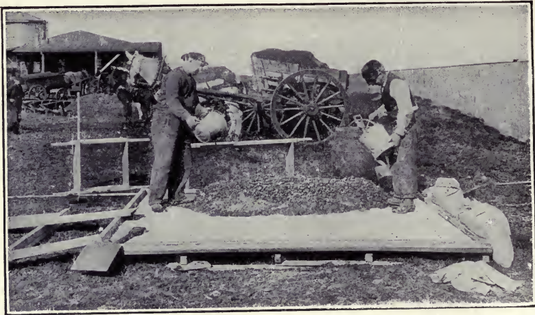
Fig. 9.—Placing the Water on the Stone (or Gravel) which is on Top of the Mixed Sand and Cement.
