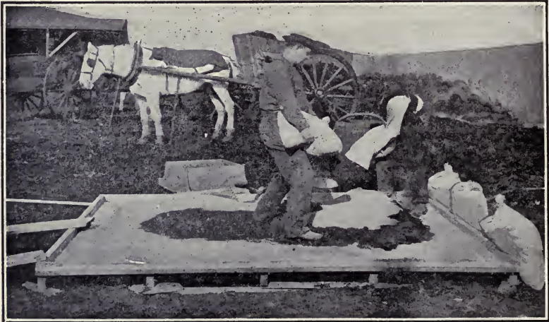
Fig. 3.—Lifting off the Sand Measuring Box and Getting Cement Ready.
