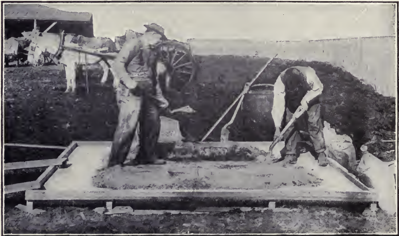
Fig. 5.—First Turning, Sand and Cement.
