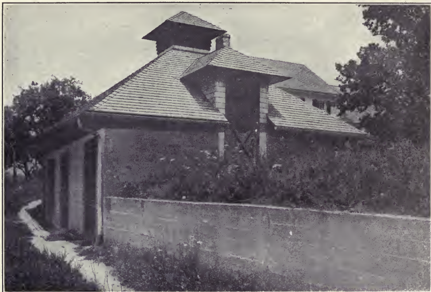
Concrete Ice House
