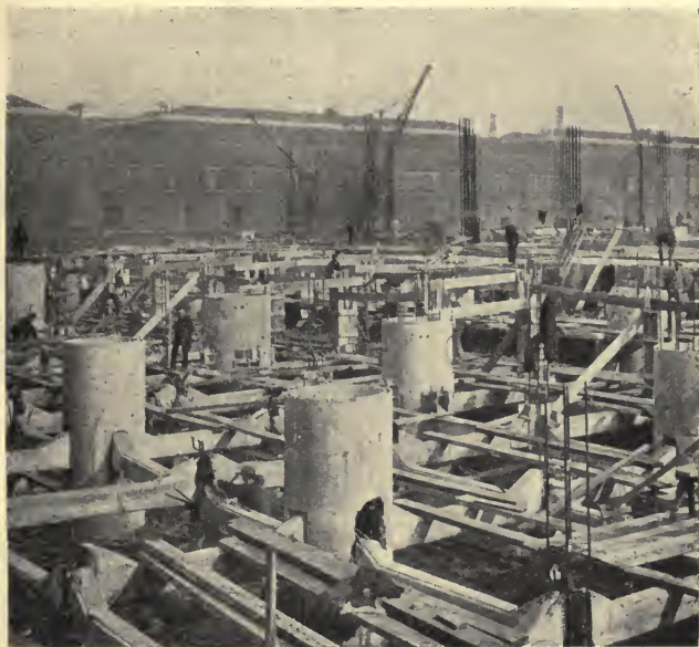
FIG. 15. CYLINDER PIERS WITH PRECAST BRACING
