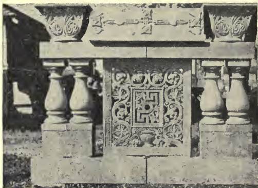
FIG. 30. MOULDED CONCRETE WORK
