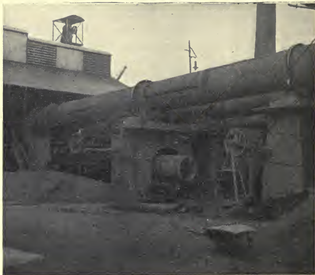
FIG. 6. ROTARY KILNS, SOUTHAM CEMENT WORKS, RUGBY
