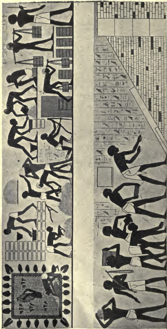
ANCIENT EGYPTIAN CONCRETE WORK, 1950 B. C.
