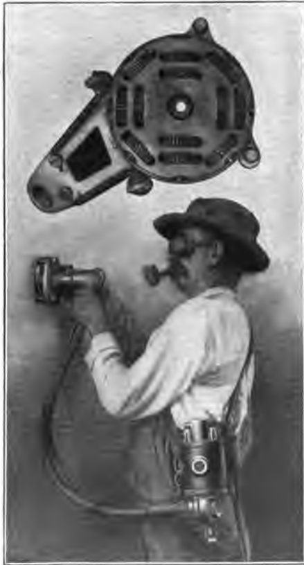
Fig. 88. Power-Driven Hand Tool for Surfacing Concrete Courtesy of "Scientific American"
