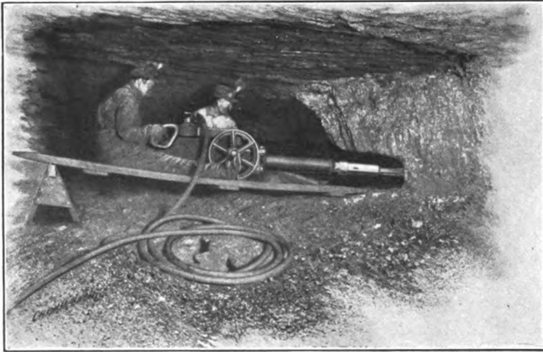
FIG. 163.—Sullivan Coal Pick, Working in a Thin Vein.
