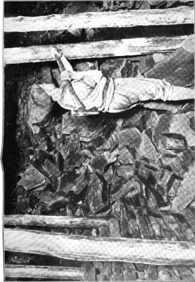
Fig 6.—A Deputy Drawing Timber near the Fallen Goaf.
