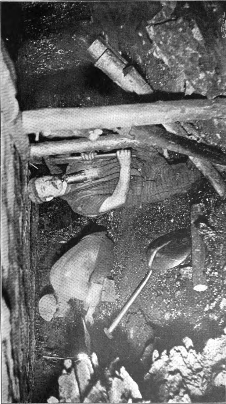
Fig. 7.—A Hewer "kirving" in a Thin Seam, and a Deputy Setting Timber.
