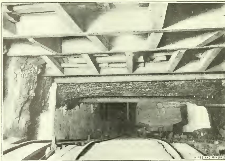
FIG. 9. CAR HAUL HANDLING EMPTIES AT FOOT OF SHAFT
