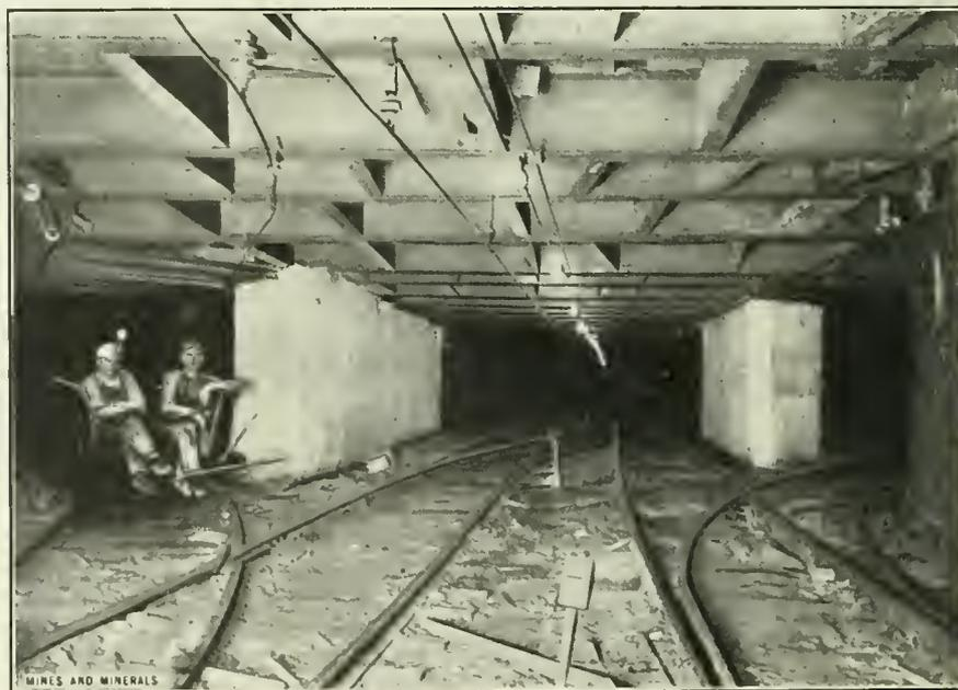
FIG. 8. TIMBERING AND CONCRETE WALLS AT TRACK INTERSECTION
