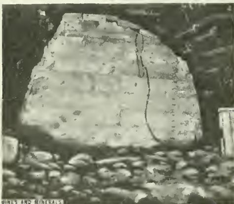
FIG. 3. SHIP-LAP PLASTERED STOPPING
