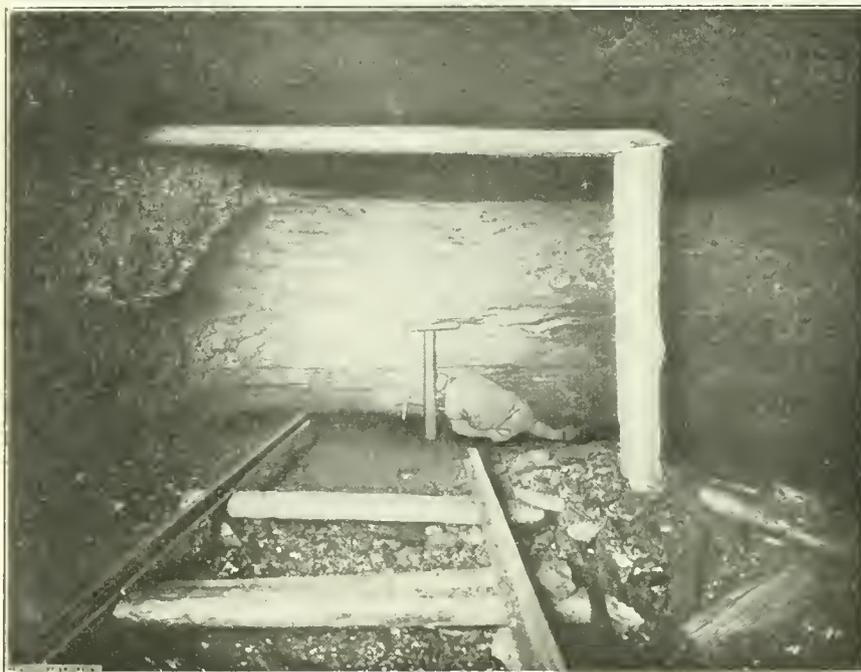
FIG. 1. FACE OF ROOM SHOWING SPRAG AND TIMBERING
