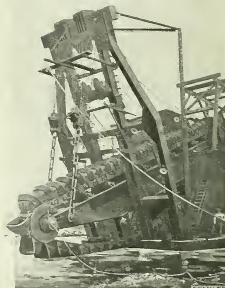
FIG. 3. LOWER TUMBLER AND BUCKET LINE, 13-FOOT DREDGE
