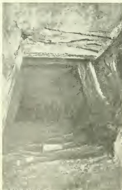
VIEW DOWN INCLINE. NOTE REGULARITY OF SECTION, THE STEPS, AND MUD-PLASTERED VENTILATING PIPES AT RIGHT
