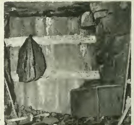
FIG. 5. BOARD STOPPING, PLASTERED
