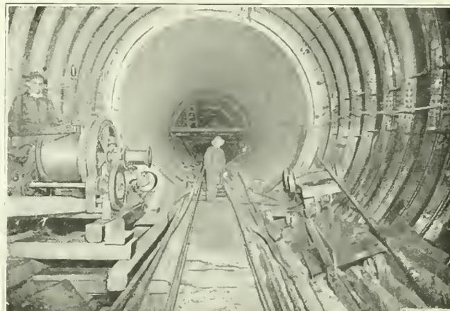
FIG. 2. RONDOUT TUNNEL, SHOWING CONCRETE AND STEEL LINING
