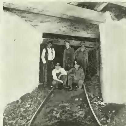
FIG. 4. PATENT LATH PLASTERED STOPPING
