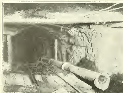
FIG. 2. SHOWING CORROSION OF PIPE
