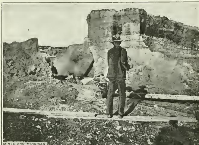
FIG. 2. BREAKING DOWN ROCK WITH HYDRAULIC NOZZLE
