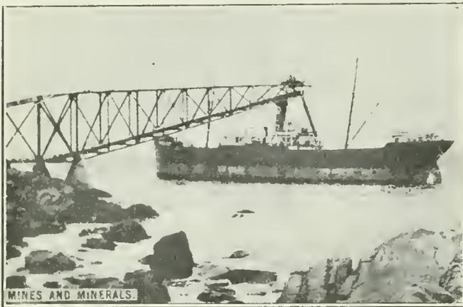
FIG. 1. ARRANGEMENT FOR LOADING ORE INTO STEAMERS
