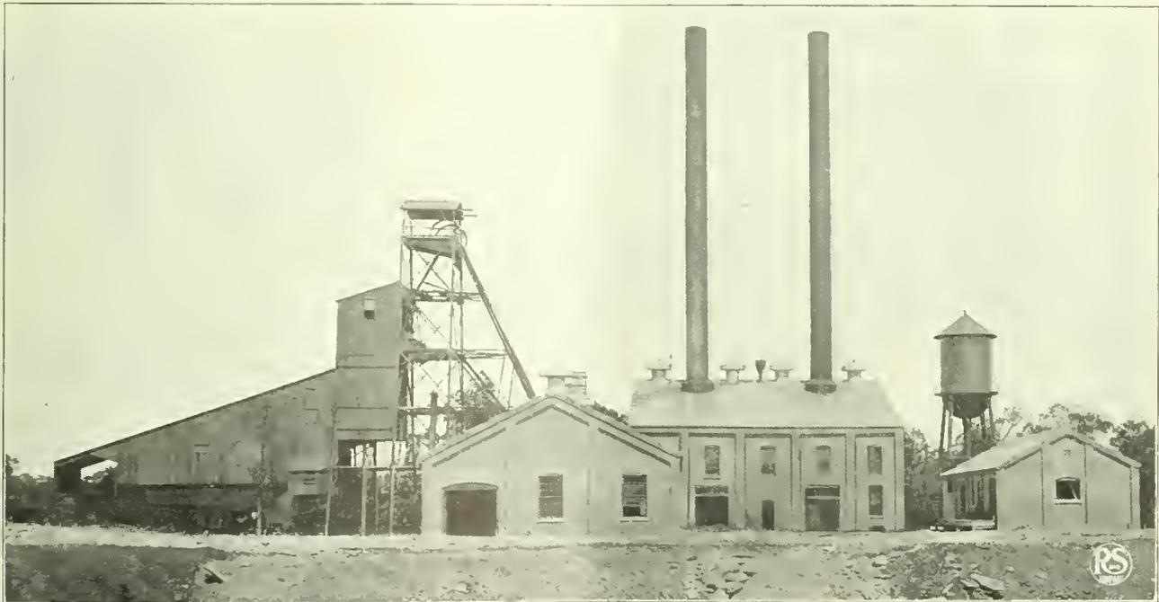
FIG. 1. BUCKNER NO. 2 MINE TIPPIE AND POWER PLANT
