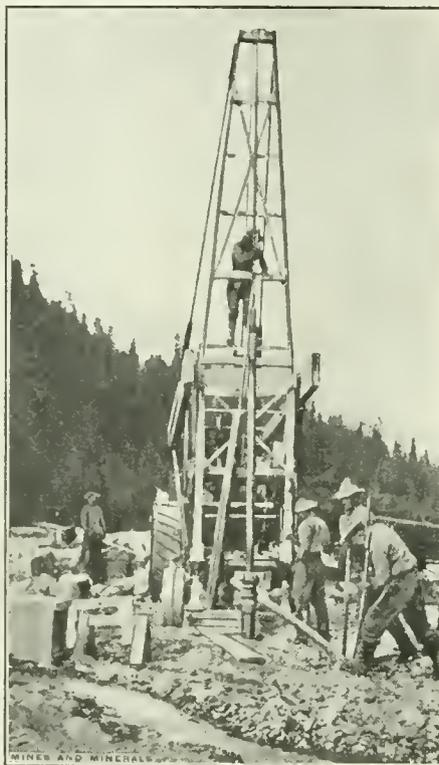
FIG. 1. DRIVING CASING
