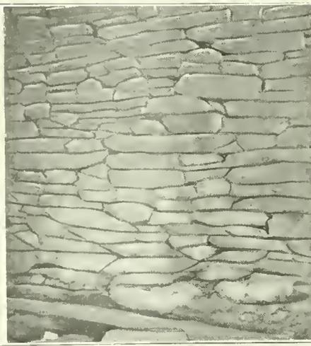
FIG. 7. SLATE STOPPING NOT PLASTERED
