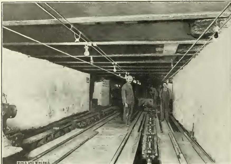
FIG. 6. PHILLIPS AUTOMATIC CAGER AND SHAFT BOTTOM
