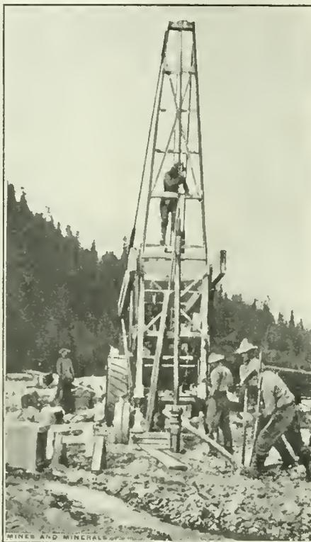
FIG. 1. DRIVING CASING
