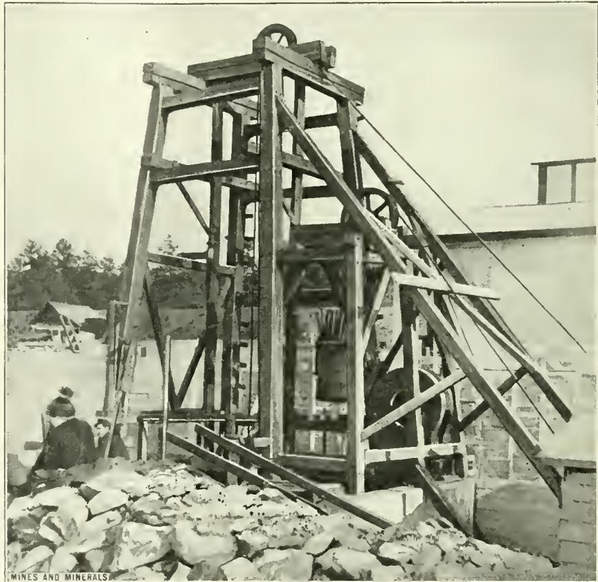
FIG 1 TEMPORARY SHAFT HEAD
