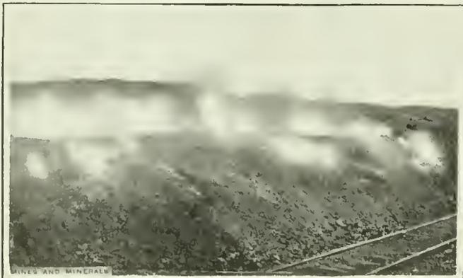
FIG. 5. HEAP OF ORE ROASTING AT COPPER CLIFF
