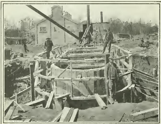
FIG. 7. FORMS IN PLACE AT VENTILATING SHAFT
