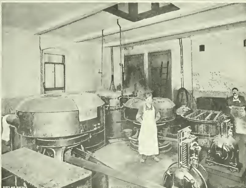
FIG. 3. WASH ROOM, SHOWING CENTRIFUGAL WASHERS
