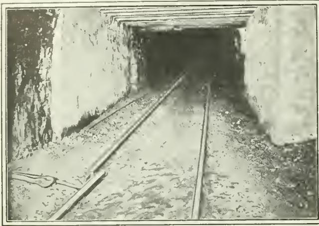
FIG. 9. SHOWING CONSTRUCTION OF OVERCAST, ALSO DERAILING SWITCH
