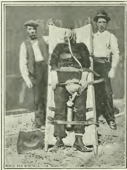
FIG. 1. MAN AND OXYGEN APPARATUS STRAPPED TO STRETCHER
