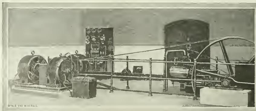
FIG. 2. MOTOR-GENERATOR SET AT CLOCK FACE COLLIERY
