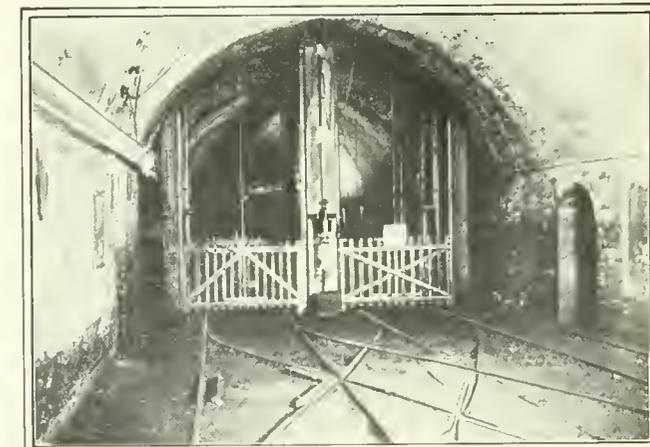
FIG. 2. GATES CLOSED AT SHAFT BOTTOM
