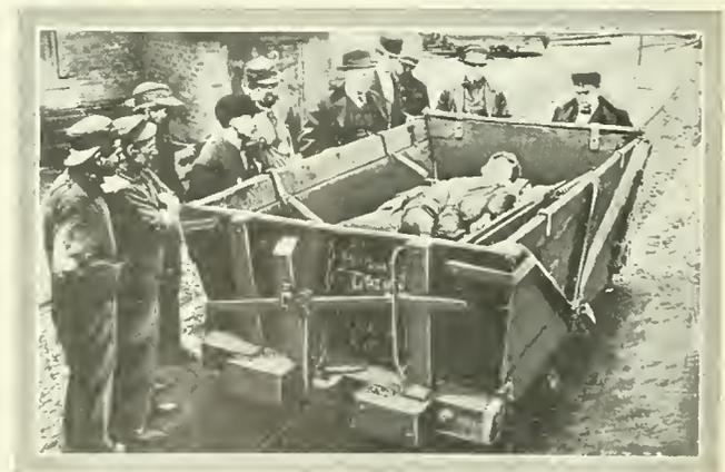
FIG. 11. HANGERS FOR STRETCHER IN MINE CAR
