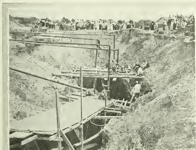
FIG. 4. RESULT OF INDISCREET DRIFTING
