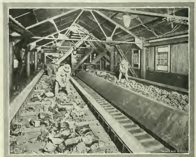
FIG. 9. PICKING BAND AND WASTE CONVEYER
