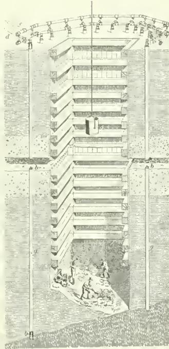
FIG. 1. SINKING IN FROZEN GROUND
