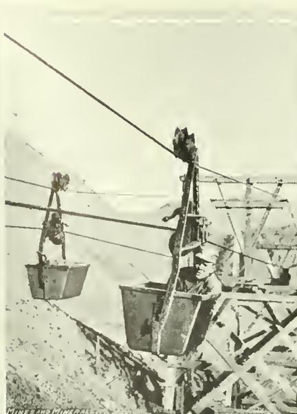
FIG. 3. BUCKET FOR PASSENGERS AND ORE
