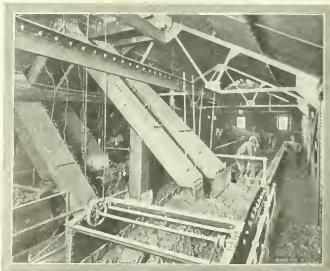
FIG. 12. CLOSED CHUTES DISCHARGING ON PICKING BAND
