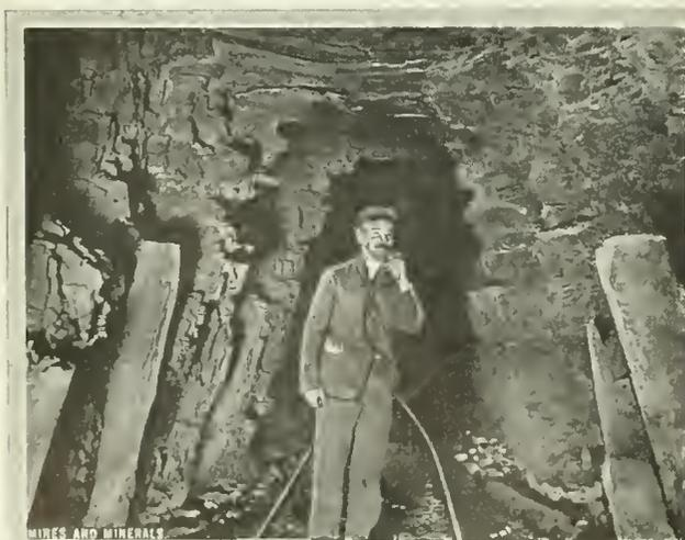
FIG. 3. ENTRY WITH COLLARS REMOVED AFTER ARCHING
