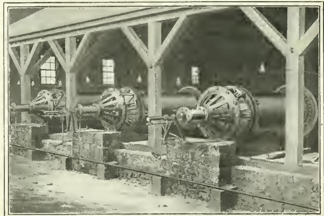
FIG. 5. BATTERY OF REVOLVING FILTERS AT EL ORO
