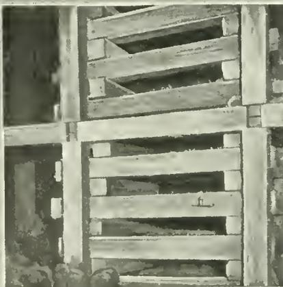
FIG. 5. CRIBBING IN STOPE, SIOUX CONSOLIDATED MINE
