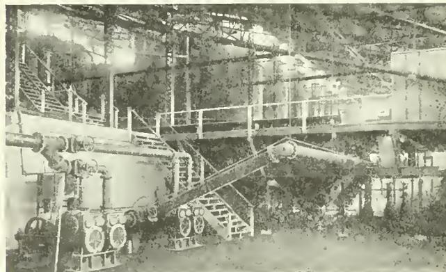
FIG. 4. VACUUM PUMPS AND ENDS OF FILTER BOXES
