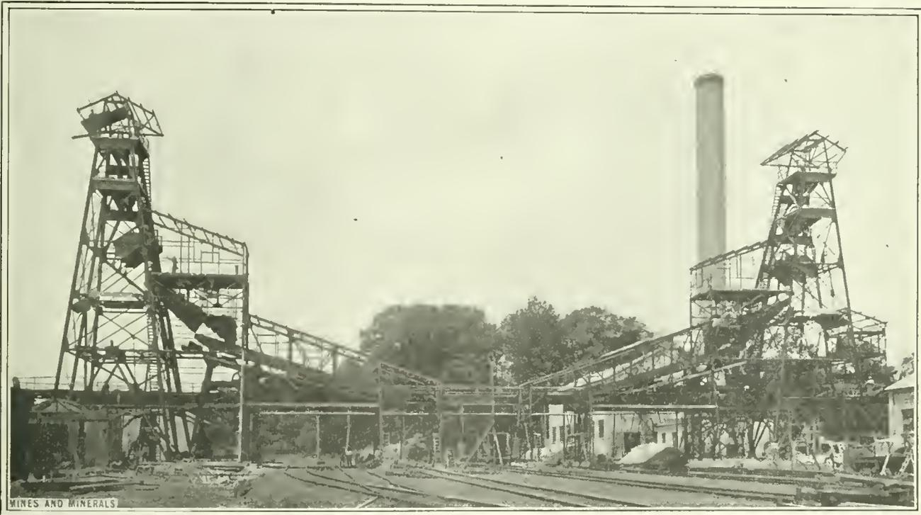
FIG. 1. TWIN TIPPLES BEFORE COVERING, UNIVERSAL MINE
