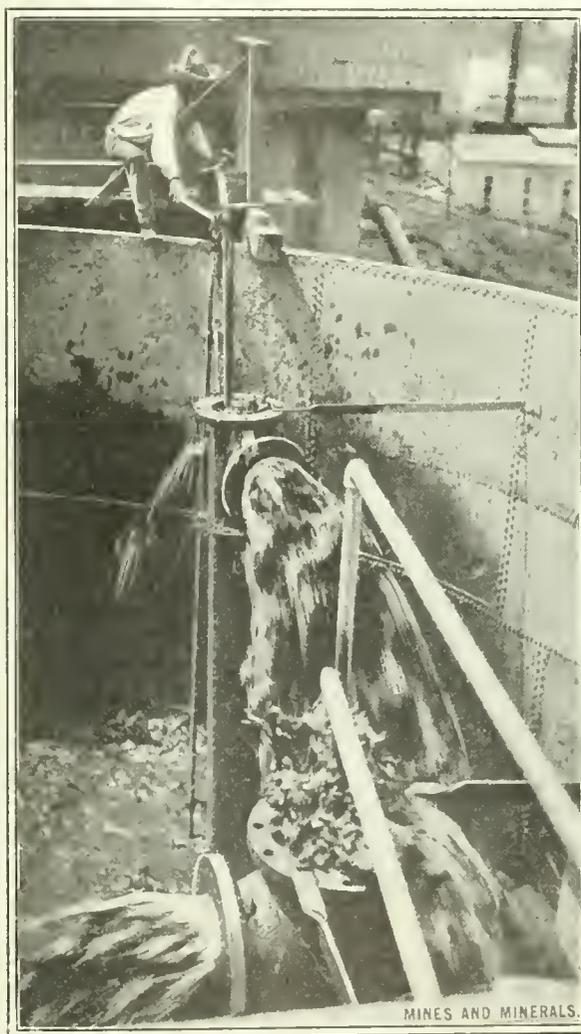
FIG. 1. TRANSFER PIPES IN TANK
