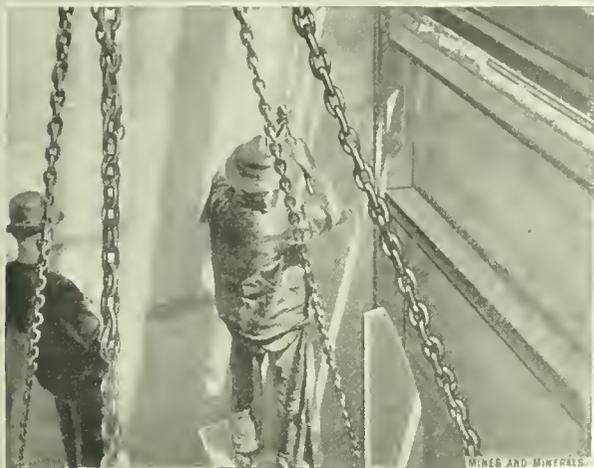
FIG. 2. DRESSING THE CONCRETE FIREPROOFING
