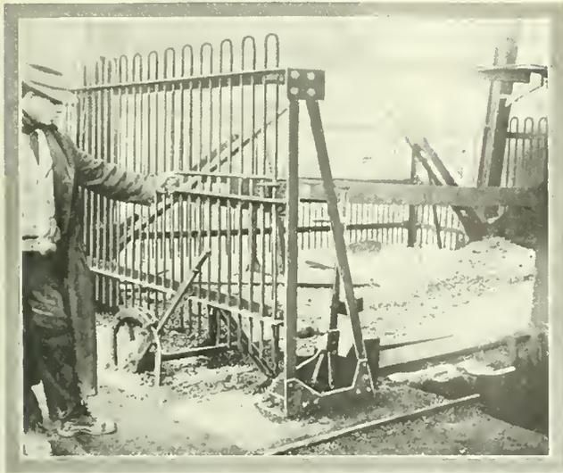
FIG. 9. SHAFT GATE LOCKING DEVICE
