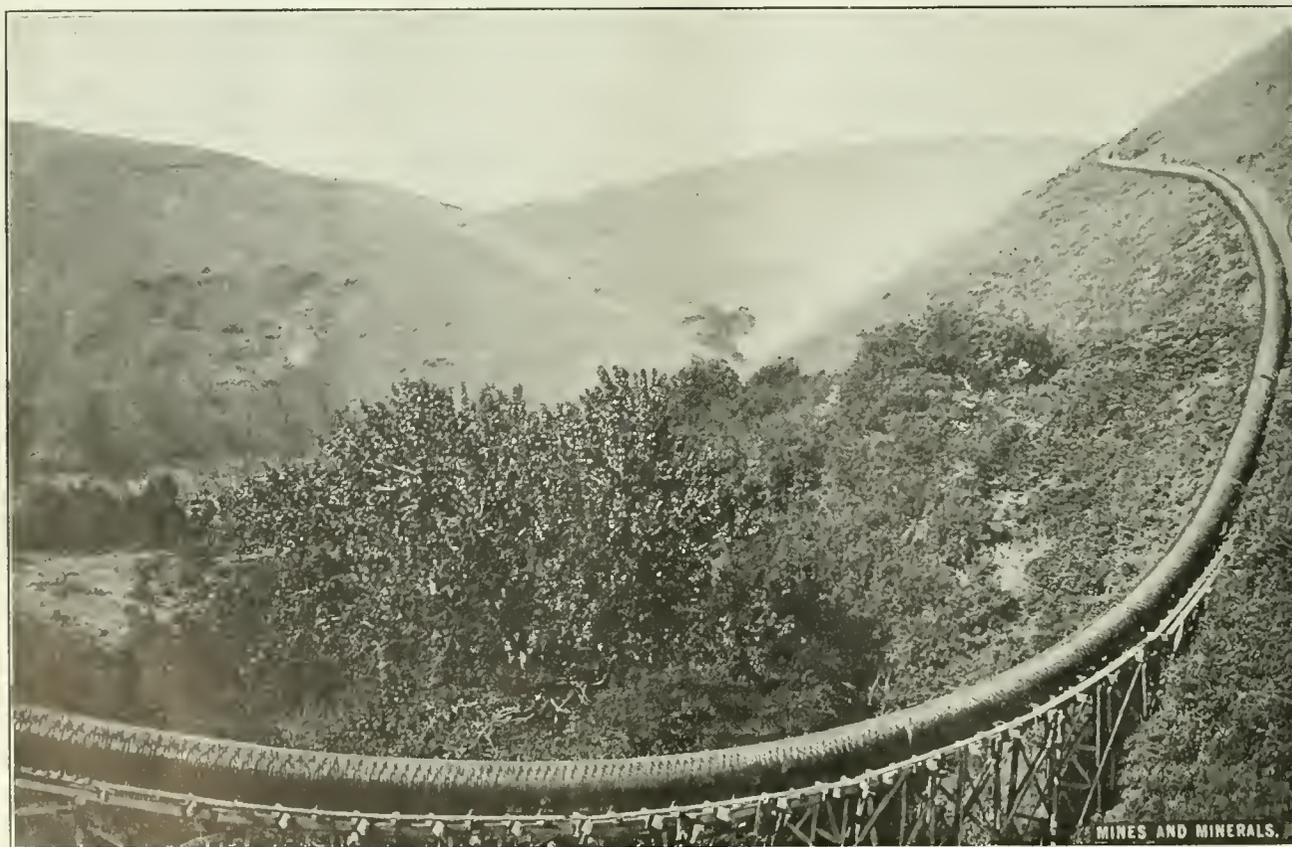
FIG. 1. CONTINUOUS WOODEN-STAVE PIPE, 5 MILES LONG, 48 INCHES DIAMETER
