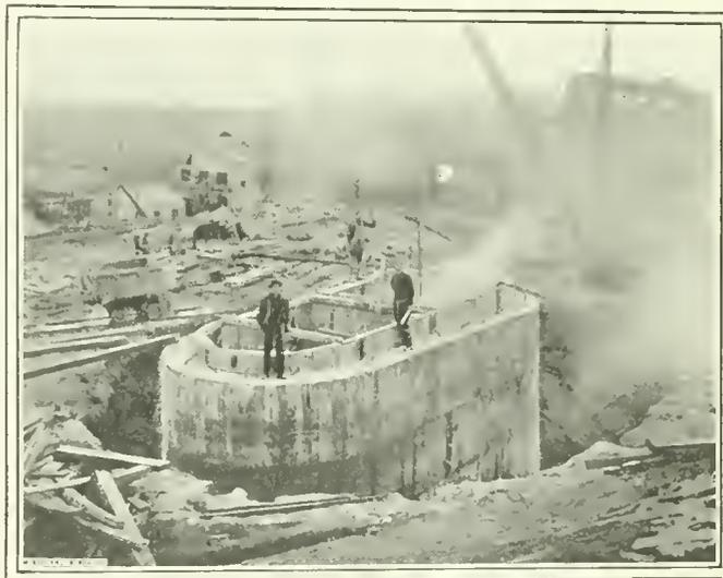
FIG. 5. VENTILATING SHAFT, CONCRETE IN PLACE BEFORE SETTLING
