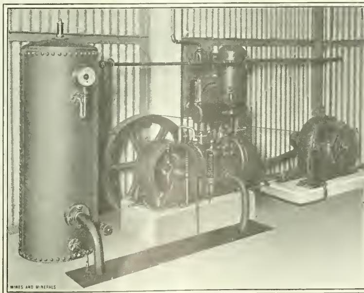
FIG. 2. ELECTRIC DRIVEN COMPRESSOR
