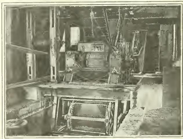
FIG. 2. EDISON 4'  $\times$  3' ROLLS AND CONVEYER
