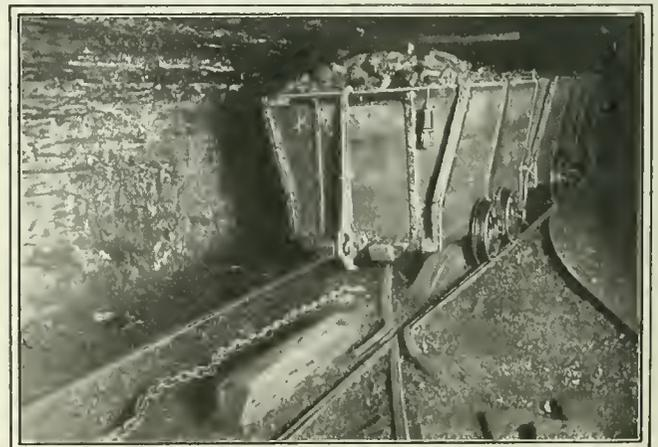
FIG. 5. NEW ARRANGEMENT FOR RELEASING TAIL-ROPE
