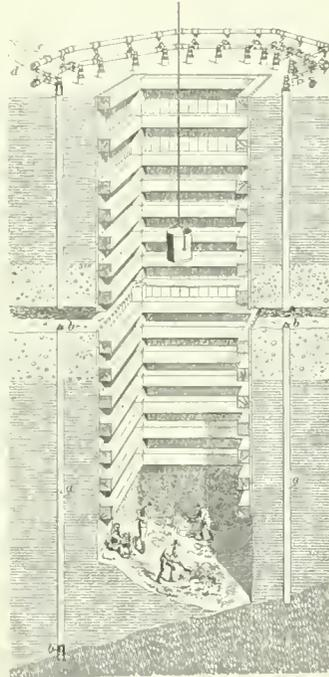
FIG. 1. SINKING IN FROZEN GROUND
