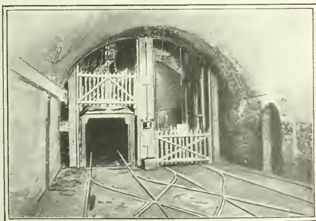
FIG. 1. CAGE AT SHAFT BOTTOM, GATE OPEN
