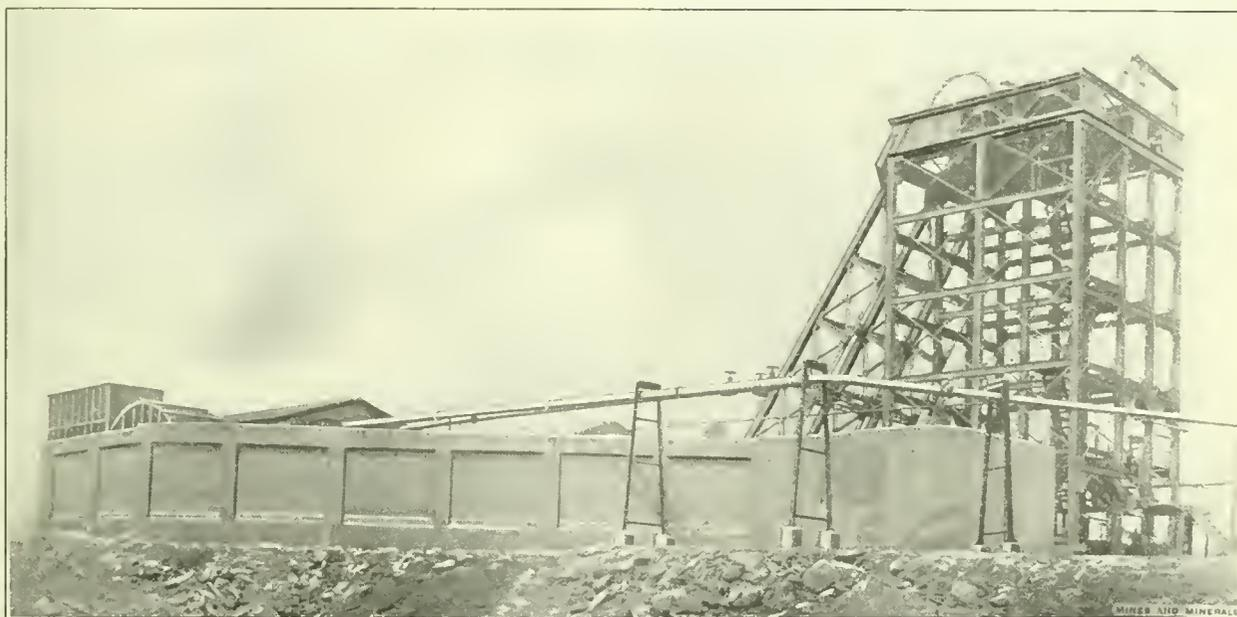
FIG. 1. FAN, AIRWAY, AND HEAD-FRAME, WOODWARD NO. 3 SHAFT
