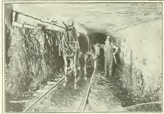
FIG. 8. SHOWING CLEARANCE ON SIDE OF GANGWAY
