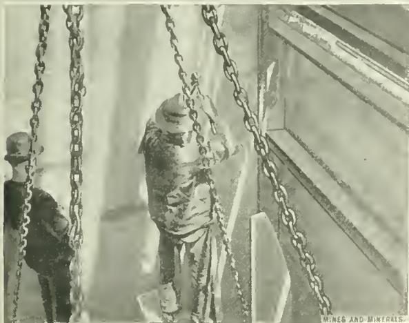
FIG. 2. DRESSING THE CONCRETE FIREPROOFING
