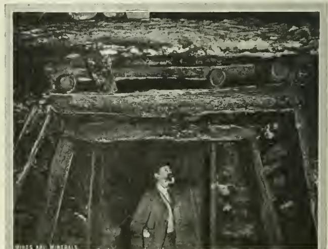
FIG. 4. TIMBERS AND LAGGING SHOWING FUNGUS GROWTH
