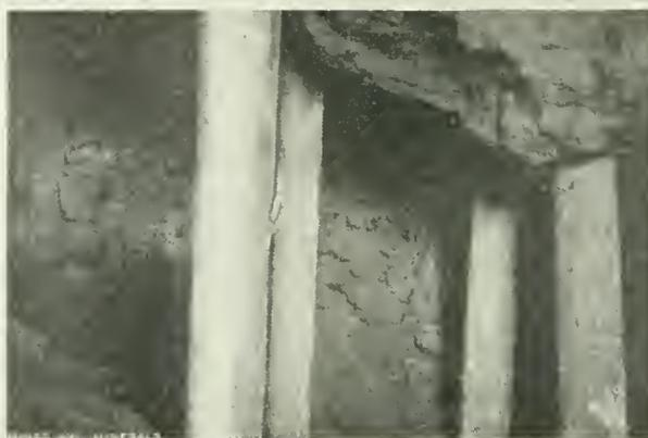
FIG. 4. HORSE OF ROCK SUPPORTED ON POSTS, FILLED SETS IN BACKGROUND
