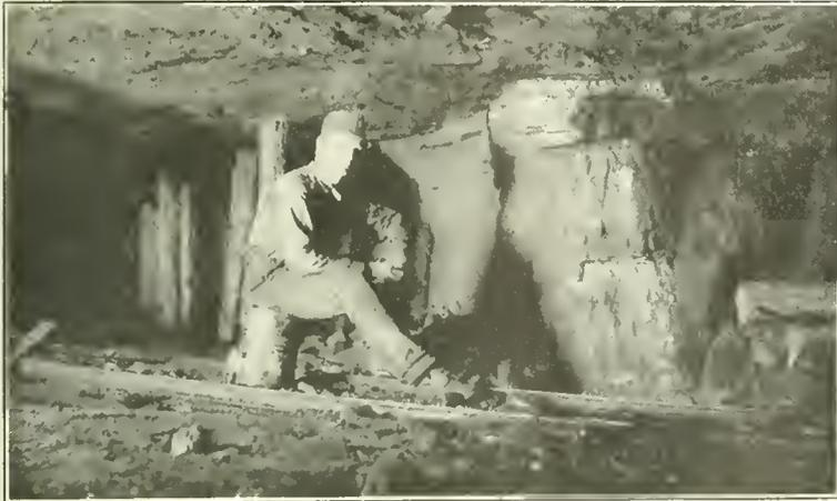
FIG. 3. SIDE OF ROOM NECK, SHOWING PROPS
