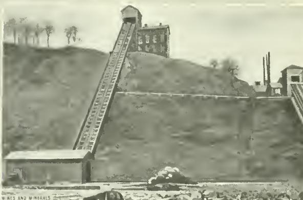
FIG. 6. NO. 2, INCLINE AND SKIP-LOADING BIN
