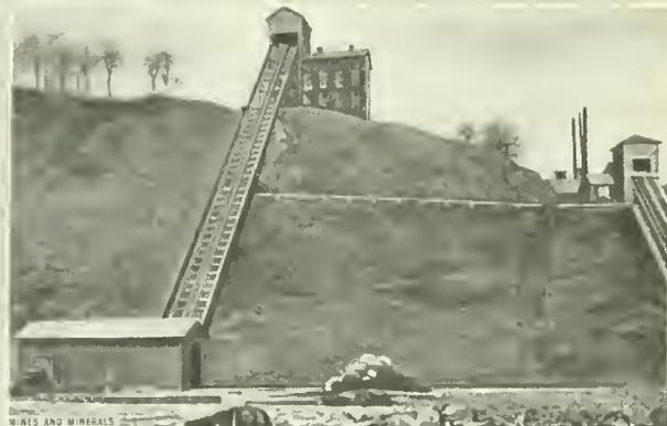
FIG. 6. NO. 2, INCLINE AND SKIP-LOADING BIN
