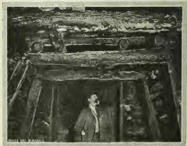
FIG. 4. TIMBERS AND LAGGING SHOWING FUNGUS GROWTH
