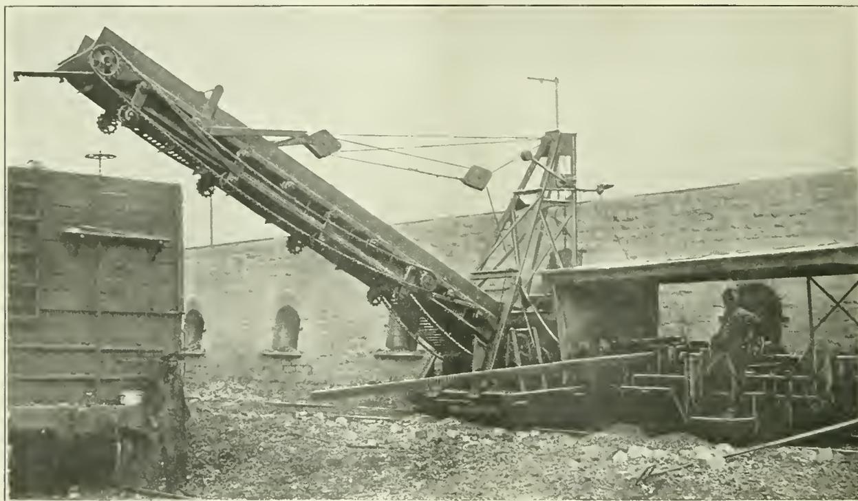
FIG. 1. ELECTRICALLY OPERATED COKE DRAWER AND LOADER
