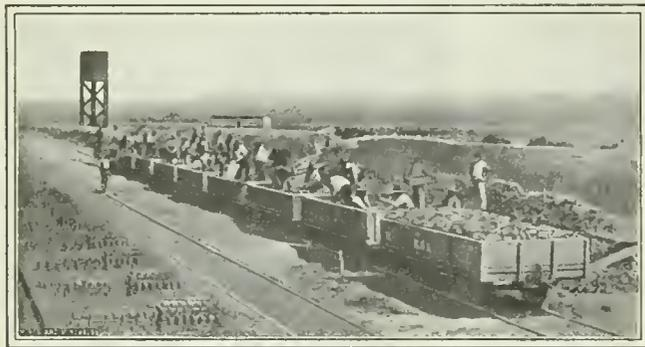
FIG. 4. HEAP ROASTING AND SINTERING NEAR BROKEN HILL
