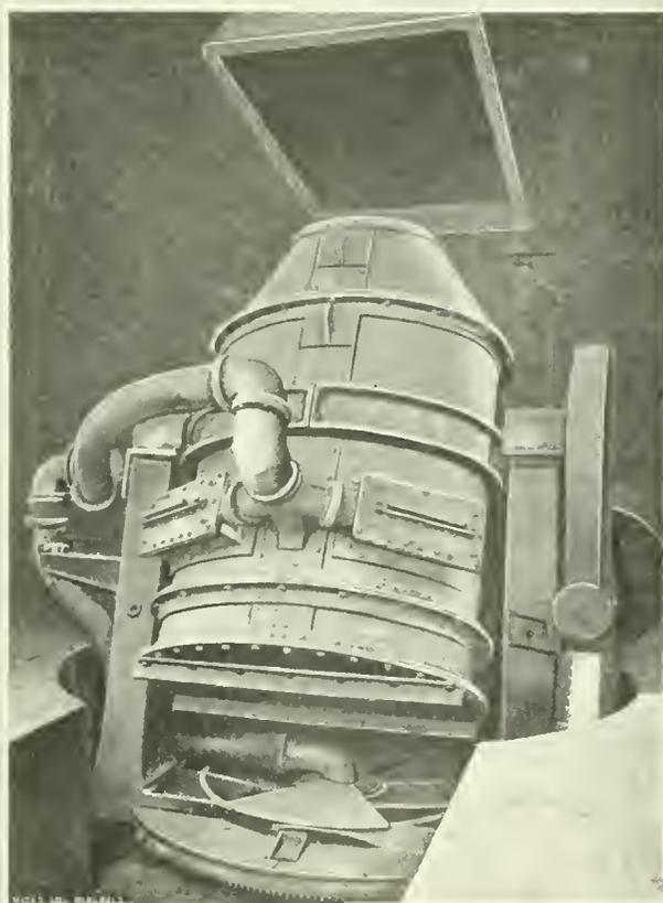
FIG. 1. OIL-FIRED CONVERTER
