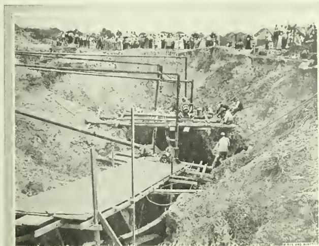
FIG. 4. RESULT OF INDISCREET DRIFTING
