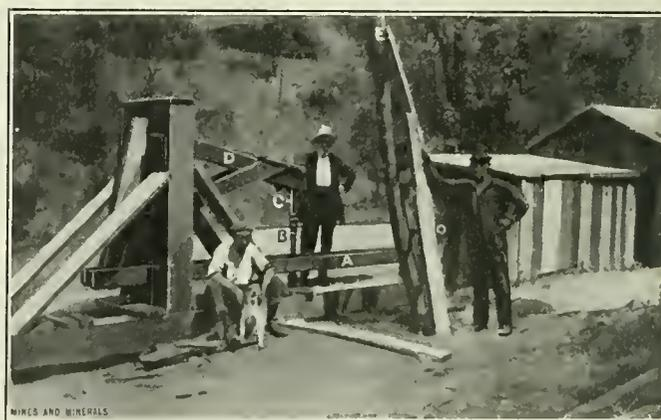
FIG. 4. HAND RIGGED PUMPING HEAD
