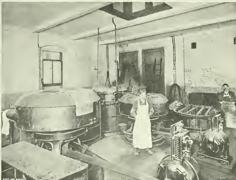
FIG. 3. WASH ROOM, SHOWING CENTRIFUGAL WASHERS
