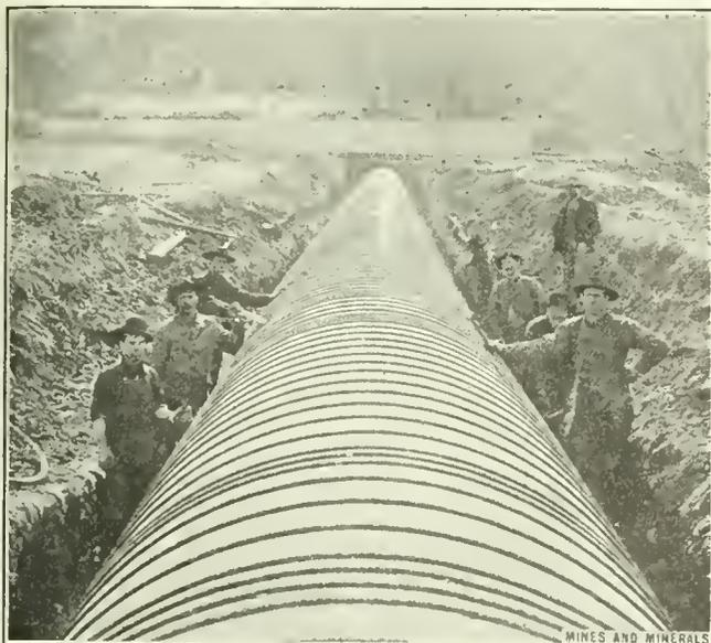
FIG. 2. WOODEN-STAVE PIPE, 86 INCHES DIAMETER
