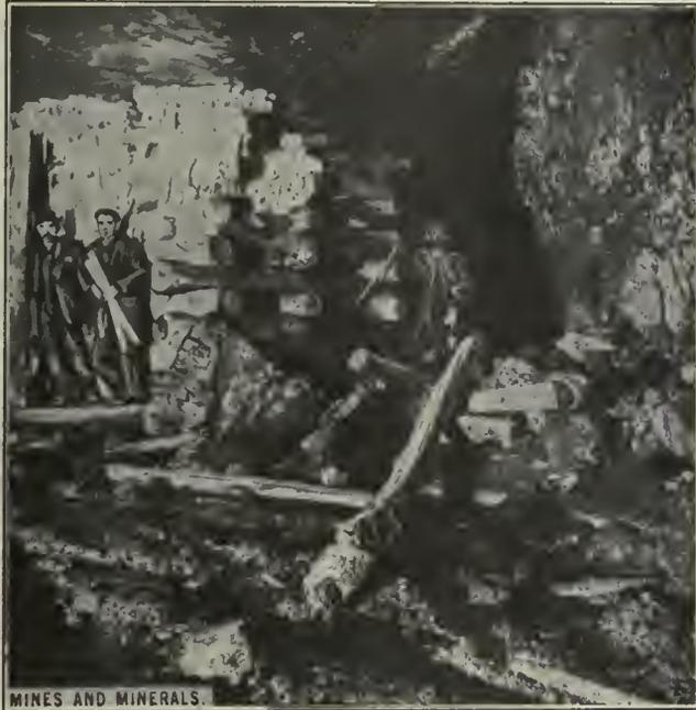
FIG. 5. FUNGI ON TIMBER CRIB
