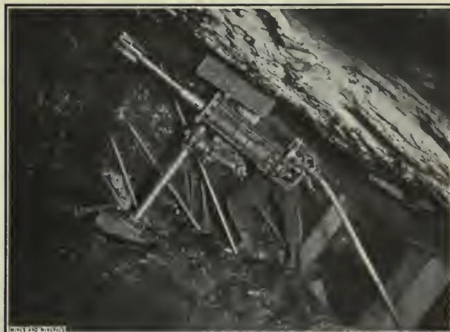
FIG. 2. CUTTING COAL WITH A NUMBER OF CHISELS IN BIT
