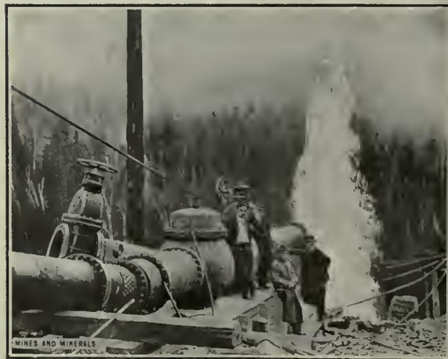
FIG. 4. AIR-PIPE VALVES AND ANCHORAGE
