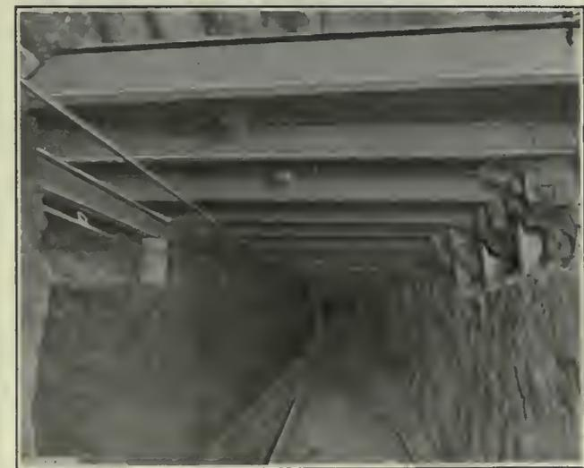
FIG. 1. STEEL MINE TIMBERS, ROBY COAL CO. DRIFT NO. 2, ADELA, O.
