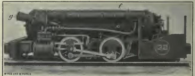
FIG. 4. LEFT-HAND SIDE OF TWO-STAGE AIR LOCOMOTIVE
