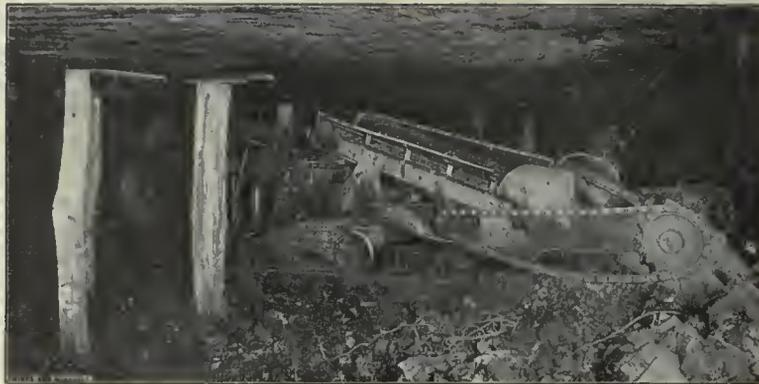
FIG. 1. COAL-LOADING MACHINE. SHOVEL MOVING INTO COAL
