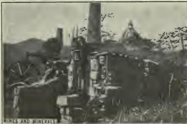
FIG. 2. AT LEFT, WATT ENGINE, PASSENGER SHAFT; IN CENTER WHAT REMAINS OF OLD CORNISH PUMP
