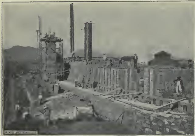
FIG. 7. CONSTRUCTING RETORT OVENS AT LAMPACITOS
