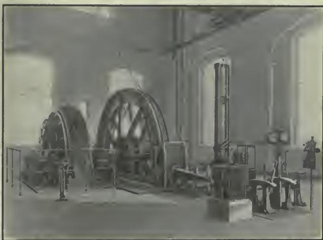
FIG. 50. ELECTRIC HOIST, KOEPE TYPE
