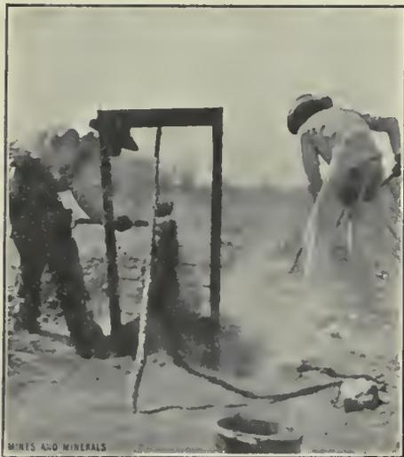
FIG. 3. USING PRIMITIVE GRIZZLY PREPARATORY TO DRY WASHING
