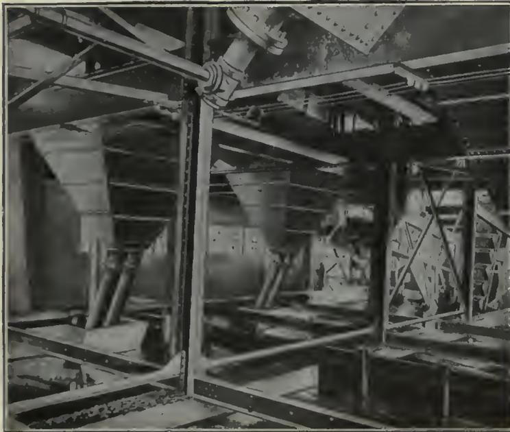
FIG. 5. HUTCHES FROM FOUR STEWART JIGS AND DISCHARGE PIPES FOR REPUSE
