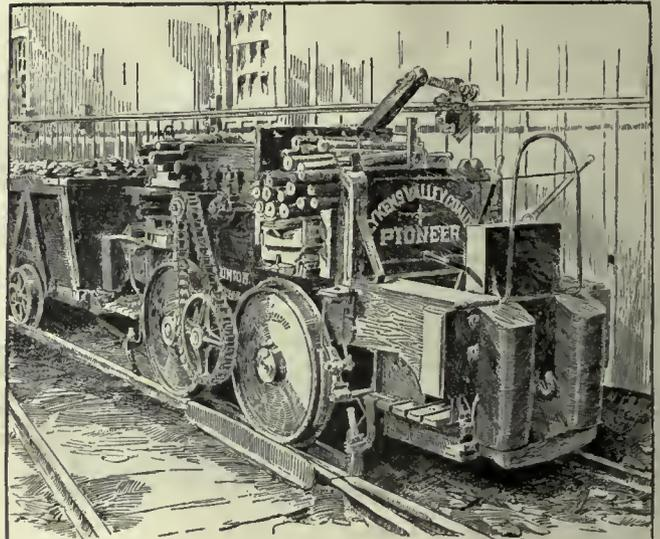
FIG. 56. FIRST ELECTRIC MINE LOCOMOTIVE USED IN AMERICA, 1887
