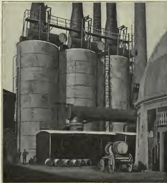
FIG. 5. AIR-DESICCATING APPARATUS
