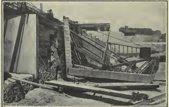
FIG. 5. MOVABLE FORMS FOR CONCRETE WORK
