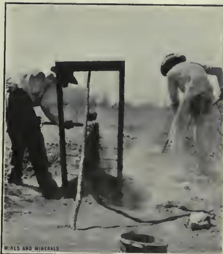
FIG. 2. SCREENING PREPARATORY TO DRY WASHING
