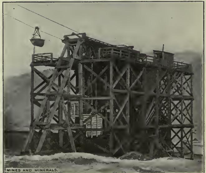
FIG. 44. LOWER DISCHARGING STATION, AERIAL TRAMWAY
