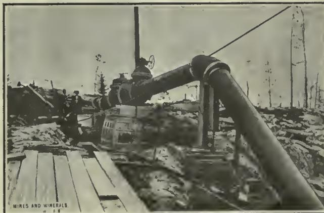
FIG. 2. AIR PIPE LINE FROM COMPRESSOR
