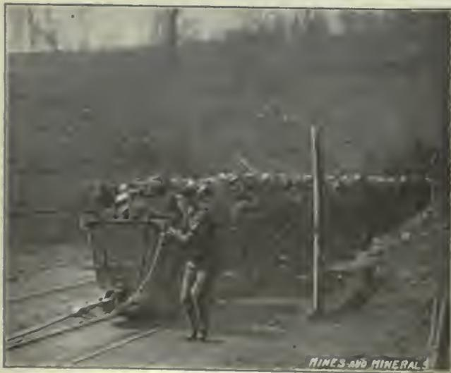
FIG. 42. CUTTING OFF CARS FROM TAIL-ROPE
