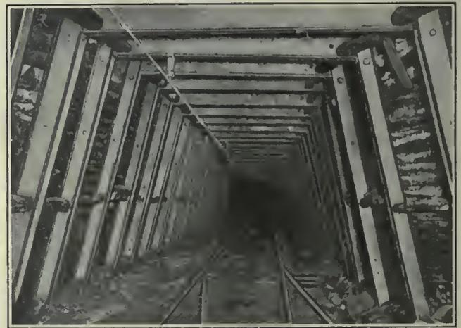
FIG. 4. THREE-PIECE STEEL SET USED BY SUSQUEHANNA COAL CO.
