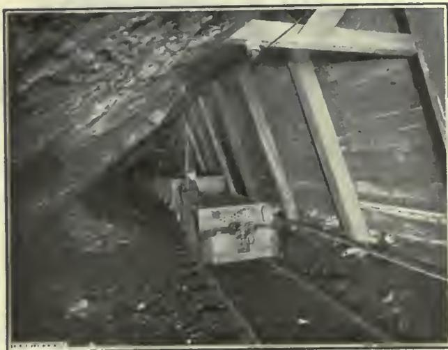
FIG. 3. HANGER ATTACHED TO TIMBER
