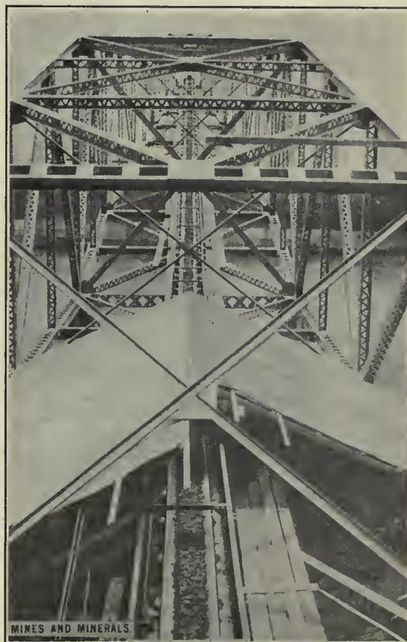
FIG. 8. CANTILEVER AND ENDLESS BELT FOR LOADING ORE
