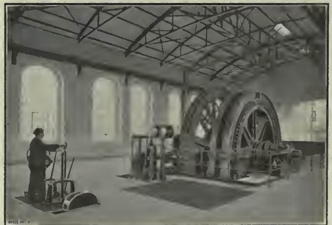
FIG. 46. ELECTRIC HOIST, KOEPE TYPE
