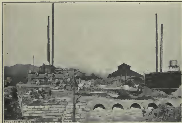
FIG. 2. RETORT COKE OVENS UNDER CONSTRUCTION AT LAMPACITOS
