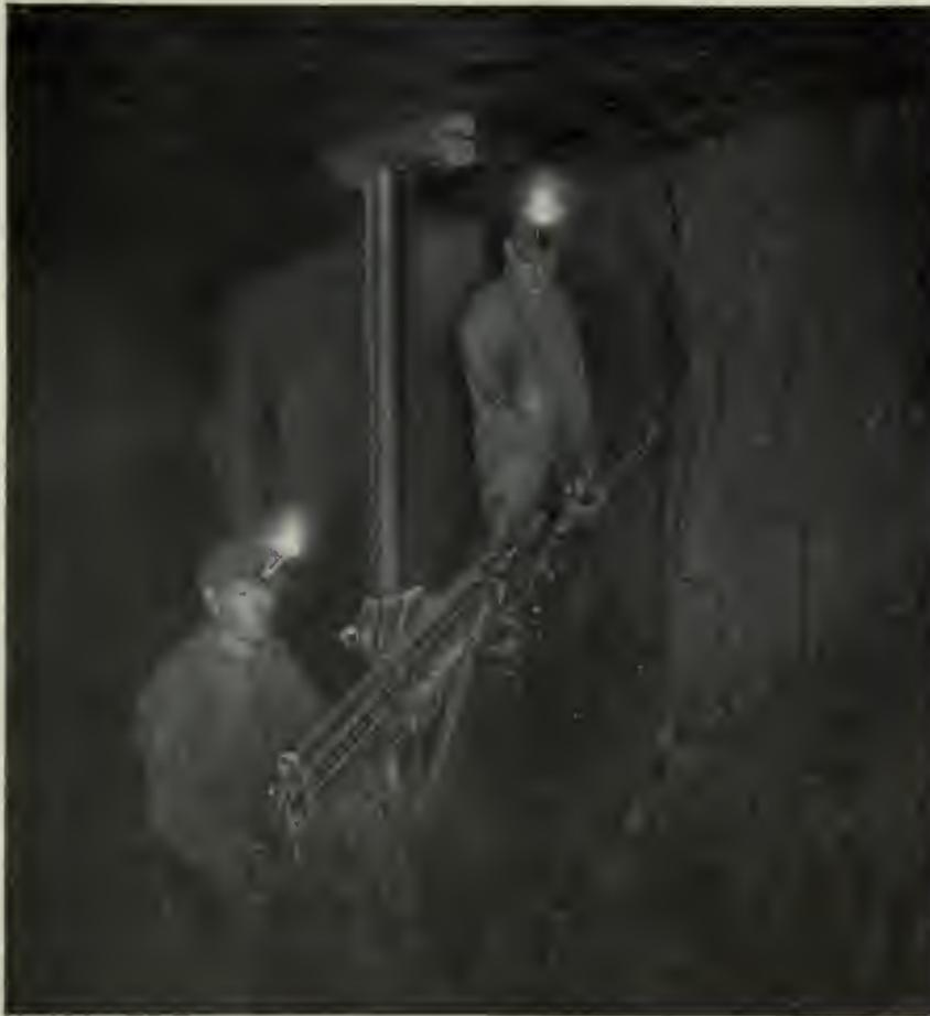
FIG. 4. DRILL IN NO. 2 MINE. SHOWING ALSO THE BLOCKY NATURE OF ORE
