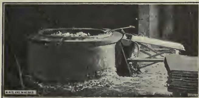
FIG. 6. CASTING MACHINE FOR LEAD CATHODES
