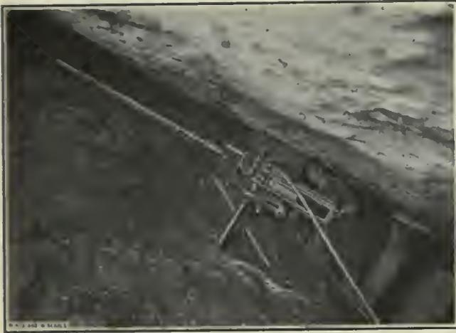
FIG. 3. POST PUNCHER USING 80-INCH EXTENSION CUTTER
