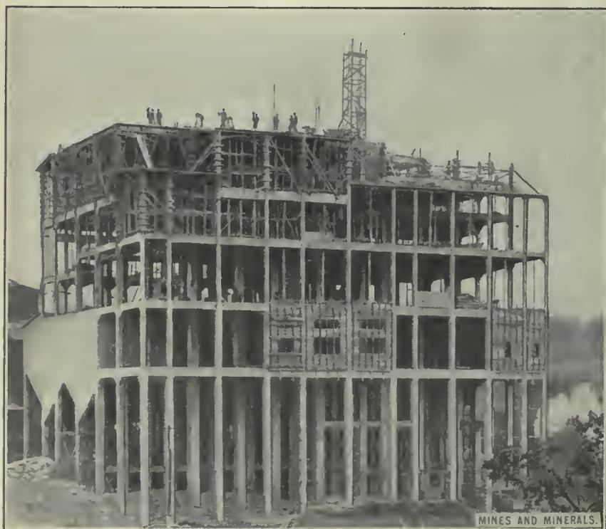
FIG. 1. TAYLOR CONCRETE BREAKER IN COURSE OF CONSTRUCTION
