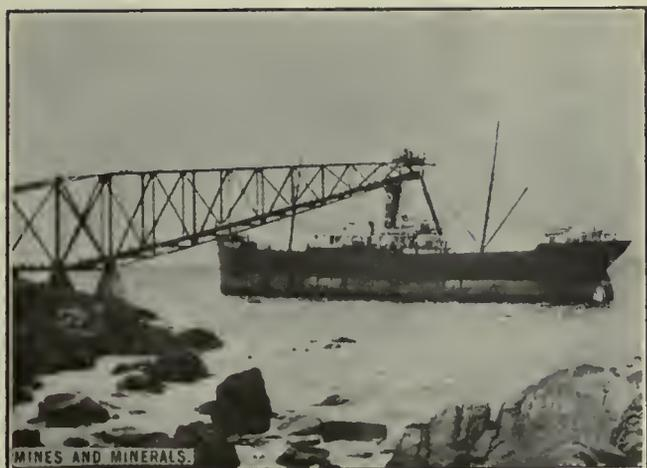
FIG. 8. ARRANGEMENT FOR LOADING ORE INTO STEAMERS
