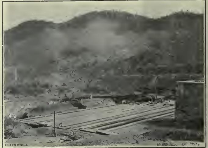
FIG. 3. "CALIFORNIAS" FOR RECOVERING COPPER FROM MINE WATERS
