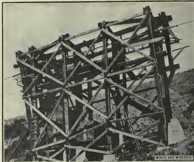
FIG. 2. TENSION STATION
