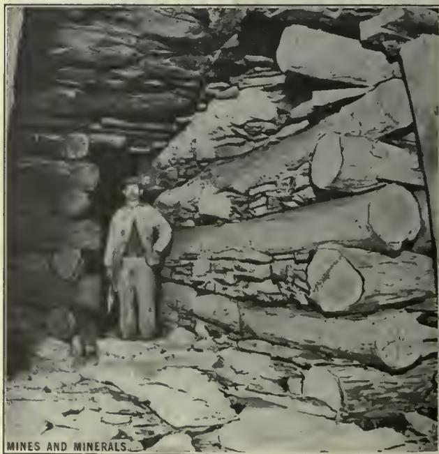
FIG. 4. TIMBER CRIB IN MINE
