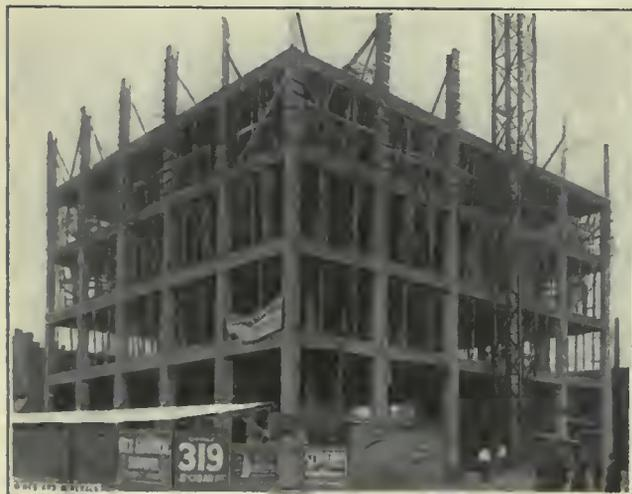
FIG. 2. CONCRETE BUILDING MADE OF ZINC TAILING
