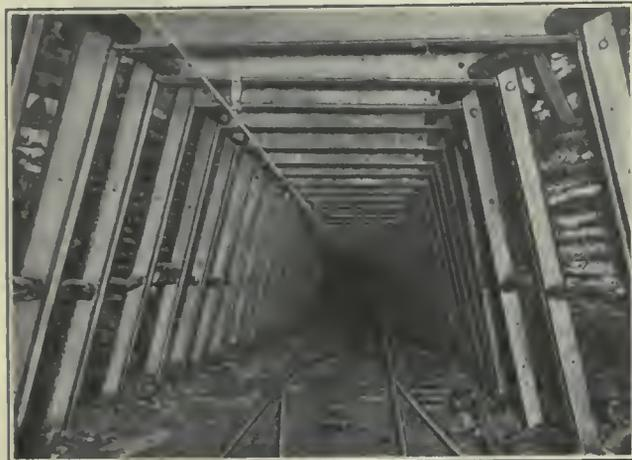
FIG. 1. THREE-PIECE STEEL SET USED BY SUSQUEHANNA COAL CO.
