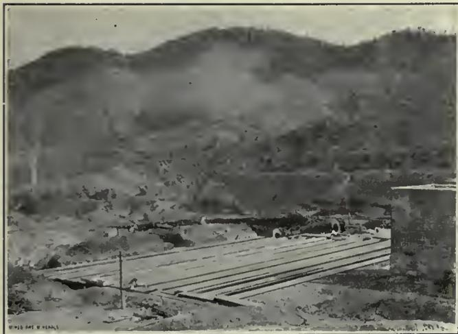
FIG. 8. "CALIFORNIAS" FOR RECOVERING COPPER FROM MINE WATERS
