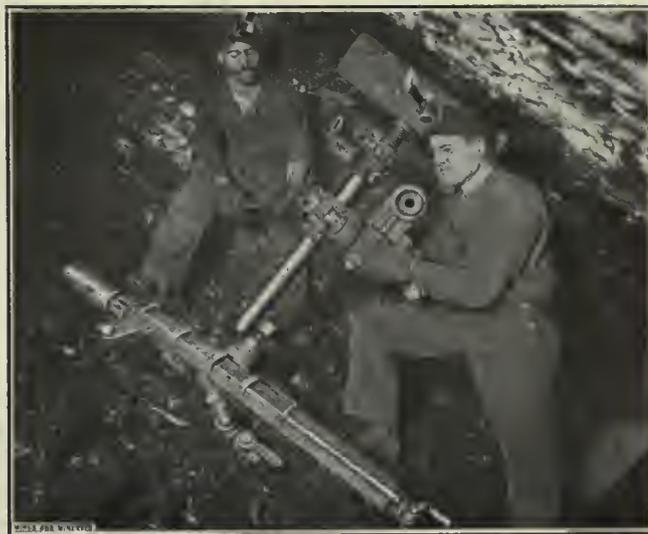
FIG. 5. SETTING UP A POST PUNCHER IN A 33-DEGREE SEAM
