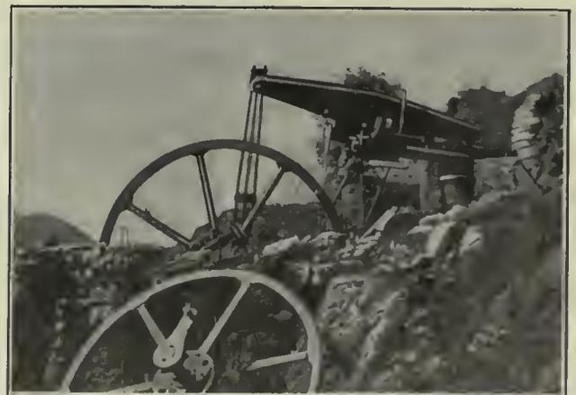
FIG. 30. WATT HOISTING ENGINE AND REEL FOR FLAT ROPE, USED IN CUBA
