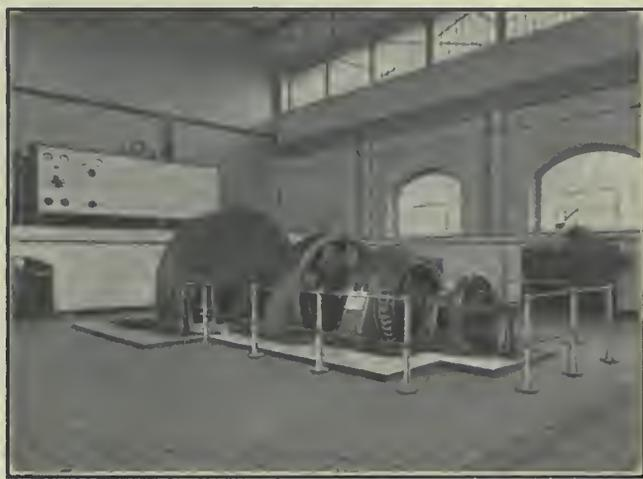
FIG. 51. ILGNER TYPE, FLYWHEEL MOTOR GENERATOR SET
