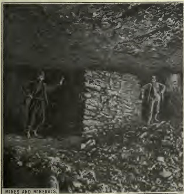
FIG. 1. DRY-MASONRY ROOF SUPPORT
