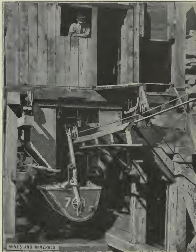
FIG. 45. LOADING STATION, AERIAL TRAMWAY
