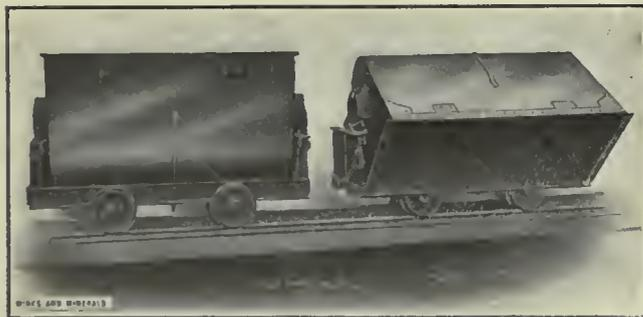
FIG. 4. ROCKER DUMP CARS USED IN TUNNEL
