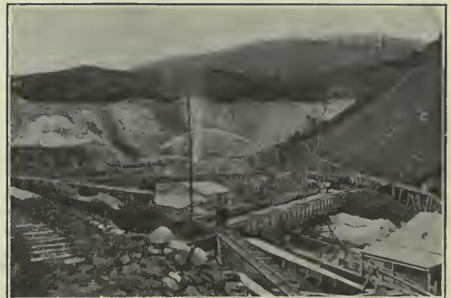
FIG. 6. OVERBURDEN AND DRIFT FACE, BRISEIS TIN MINE
