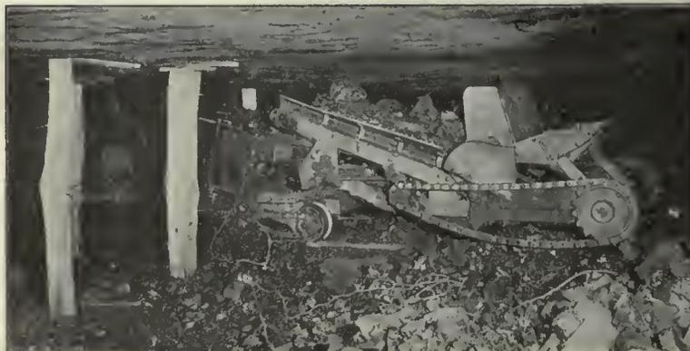
FIG. 2. COAL-LOADING MACHINE LOADING INTO CONVEYER
