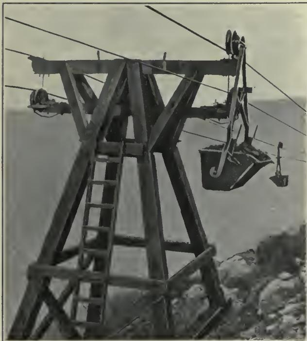
FIG. 4. LOADED BUCKET PASSING OVER TOWER SADDLE
