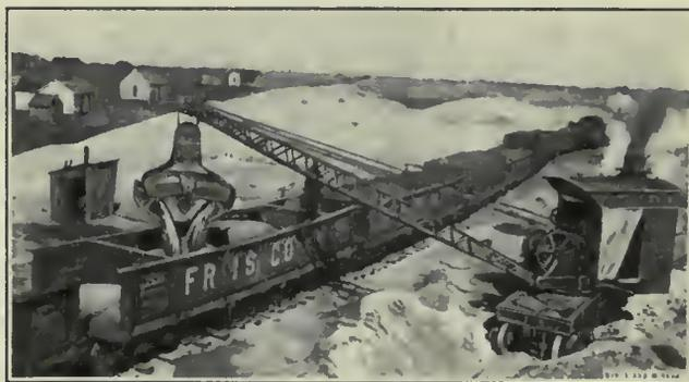
FIG. 3. LOADING TAILING FOR RAILROAD BALLAST, JOPLIN
