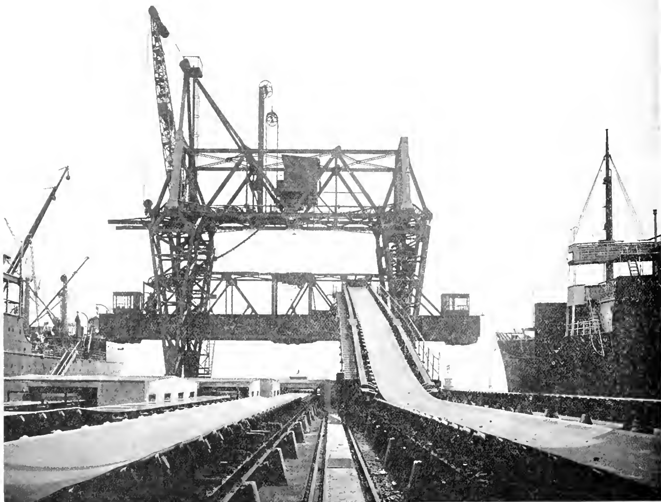
Fig. 6. The belts in use at Curtis Bay are 60 inches in width, with a capacity of 1,500 tons of coal an hour, running at 500 feet per minute. The loading tower shown in center travels along the pier in a horizontal direction and the shuttle ram (with little houses at either end for the operator) working in and out at right angles to the travel of the towers will load a hatch uniformly and reduce trimming to a minimum.
