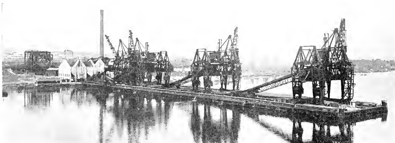
Fig. 7. View of modern dumping pier at Curtis Bay. Car dumpers are shown at left and loading towers on the pier at right. The balancing bin is interposed between the car dumpers and the pier.
