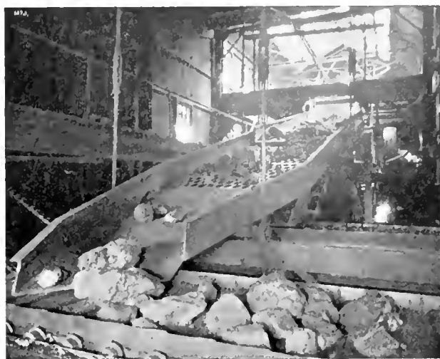
Fig. 8. Shaker Screens in Boissevain Tippie of Pocahontas Fuel Co., Pocahontas, Va., showing discharge of Lump onto Picking Table.
