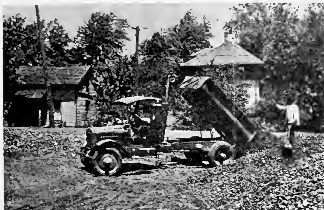
Fig. 2. Placing the First Layer of Coal on Storage Plat at the University of Illinois.
