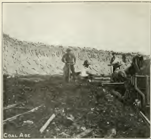
DRILLING HOLE PREPARATORY TO SHOOTING
