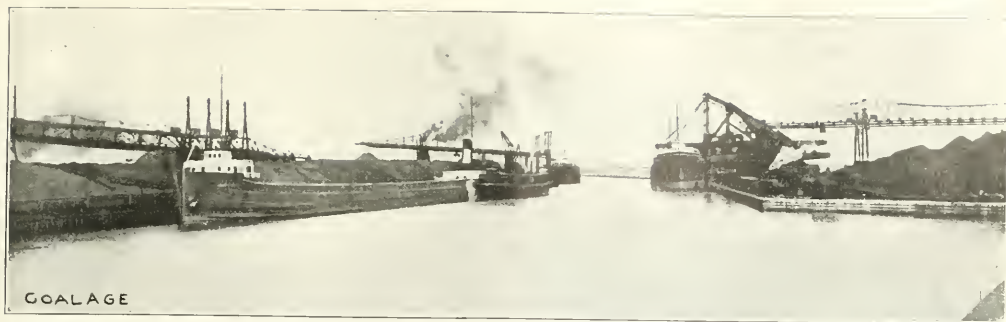
CONNEAUT HARBOR (OHIO). SHOWING TRAVELING-BRIDGE STORAGE TRAMWAYS IN THE BACKGROUND
