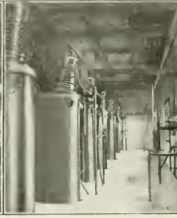
FIG. 12. SINGLE-PHASE TRANSFORMERS
