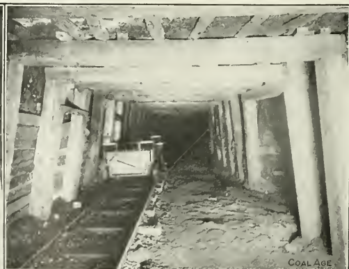
SHOWS STYLE OF TIMBERING EMPLOYED IN ENTRIES OF ROSEDALE MINE AT CALGARY
