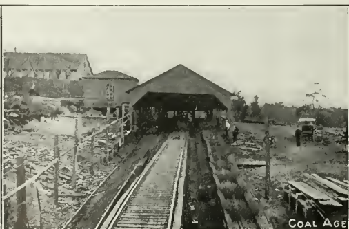
VIEW OF RODEN TIPPLE, SHOWING APPROACH TO DUMP AND EMPTIES DESCENDING
