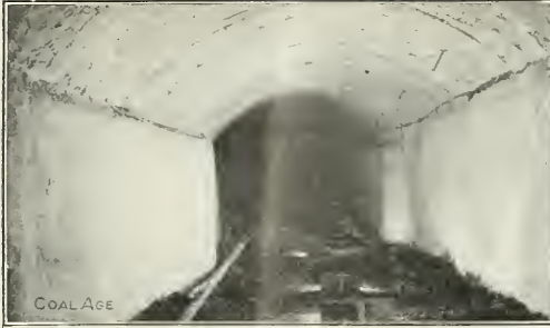
SHOWS STYLE OF CONCRETE ARCH USED NEAR FOOT OF AIR SHAFT IN MINES OF MADISON COAL CORPORATION
