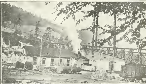
TENNESSEE'S STATE COKE PLANT. TIPPLE BINS AND WASHER ON THE LEFT AND POWER PLANT ON THE RIGHT
