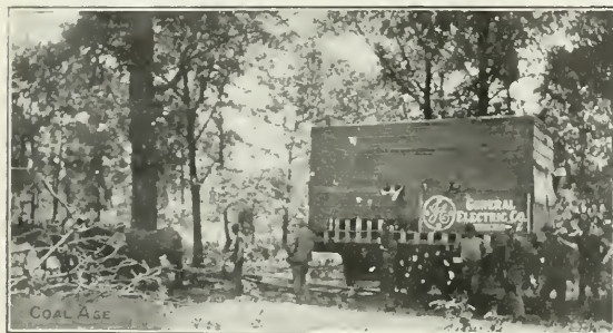
TWO VIEWS OF THE 500-KW. TURBINE BEING TAKEN THROUGH THE WOODS TO THE POWER PLANT
