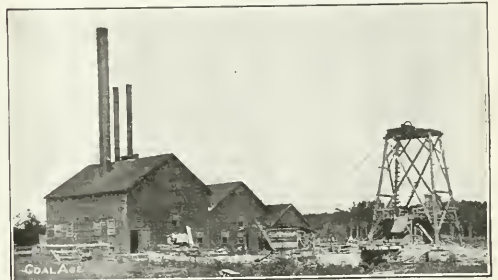
BOILER AND ENGINE HOUSE AND TEMPORARY HEADFRAME
