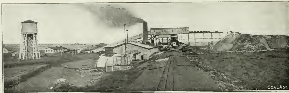
CANADA WEST COAL CO.'S PLANT, AT FABER, ALBERTA, CAN. (Produces a high grade of domestic coal, and has a capacity of 2000 tons per day.)
