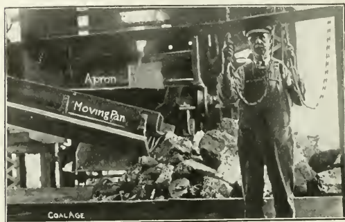
AN ILLINOIS LOADING BOOM
