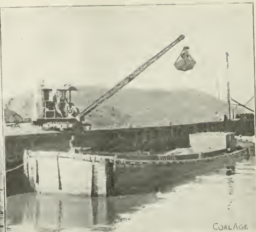
FIG. 7. UNLOADING BOATS WITH LOCOMOTIVE CRANE AND CLAMSHELL BUCKET
