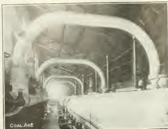
FIG. 12. STEAM HEADER AND ITS CONNECTIONS IN BOILER PLANT
