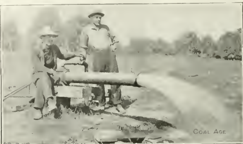
PUMPING WATER OUT OF CROWN HILL NO. 1 MINE, AT CLINTON, IND., WITH "AIR LIFT"
