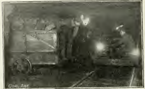
GATHERING LOCOMOTIVE HAULING LOADED CAR FROM ROOM BY MEANS OF A STEEL CABLE
