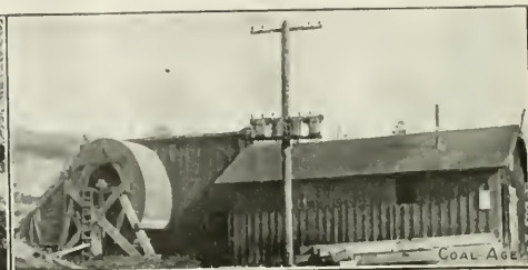
SUBSTITUTING ELECTRICITY FOR STEAM. NOTE IDLE EXHAUST PIPE
