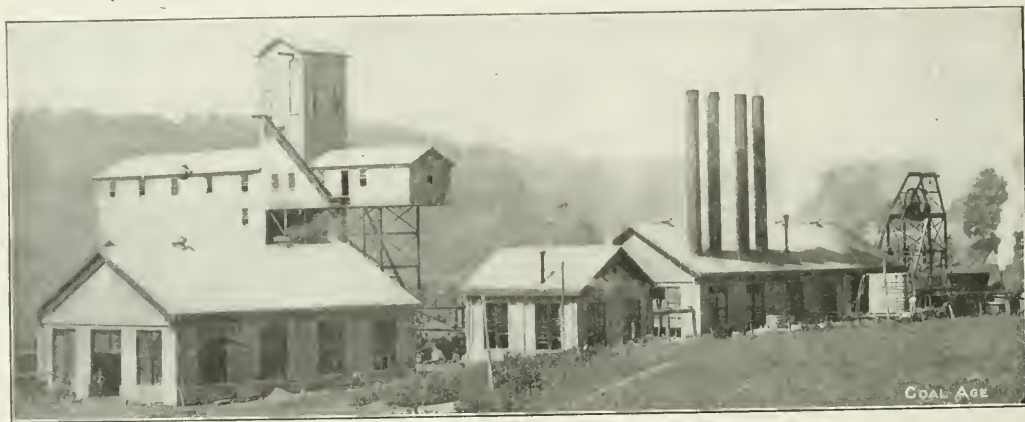
VIEW OF TIPPLE, SHOWING HOISTING-ENGINE, POWER AND BOILER HOUSES WITH MAN HOIST ON THE RIGHT
