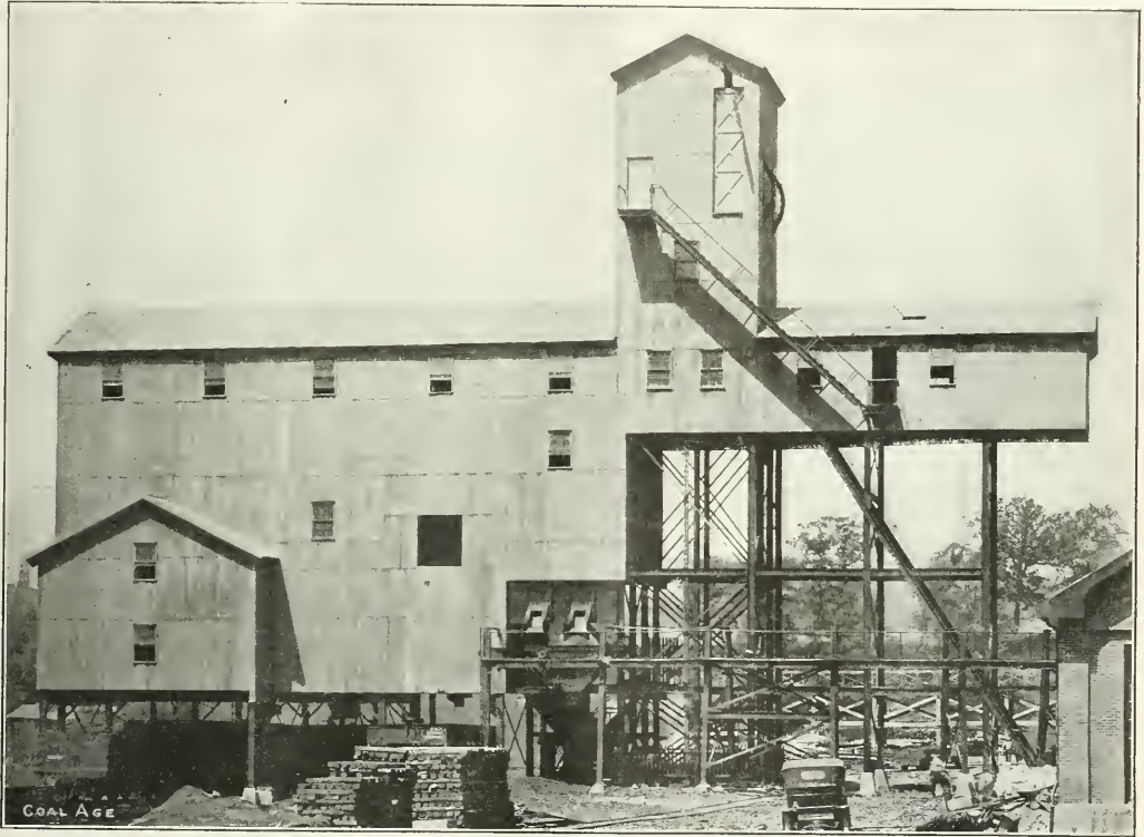
VIEW OF TIPPLE, SHOWING BOILER-COAL BIN WITH TRESTLE AND ELECTRIC LARRY
