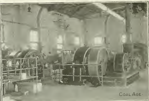
GENERATORS AT COLLIERY NO. 1
