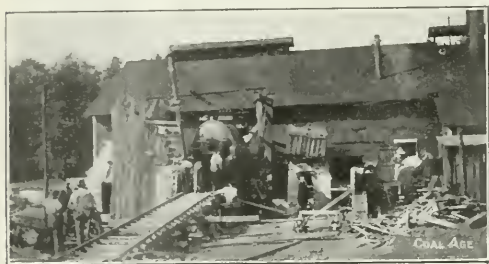
PLACING THE TURBINE ON FOUNDATION
