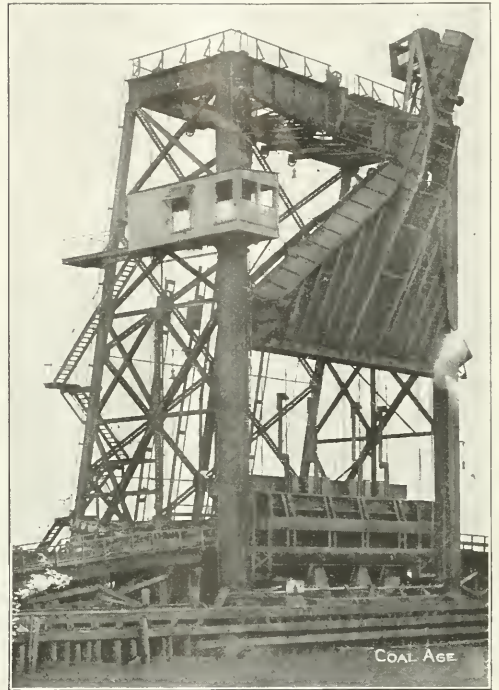
THE PITTSBURGH COAL CO.'S CAR-DUMPING MACHINE ON P. R.R. TRACKS, CLEVELAND, OHIO
