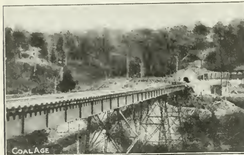
STEEL DOUBLE-TRACK INCLINE, CONNECTING TIPPLE AND MINES, RODEN COAL CO., MARVEL, ALA.
