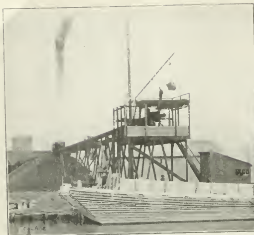
FIG. 6. UNLOADING COAL FROM BOATS WITH MAST AND GAFF
