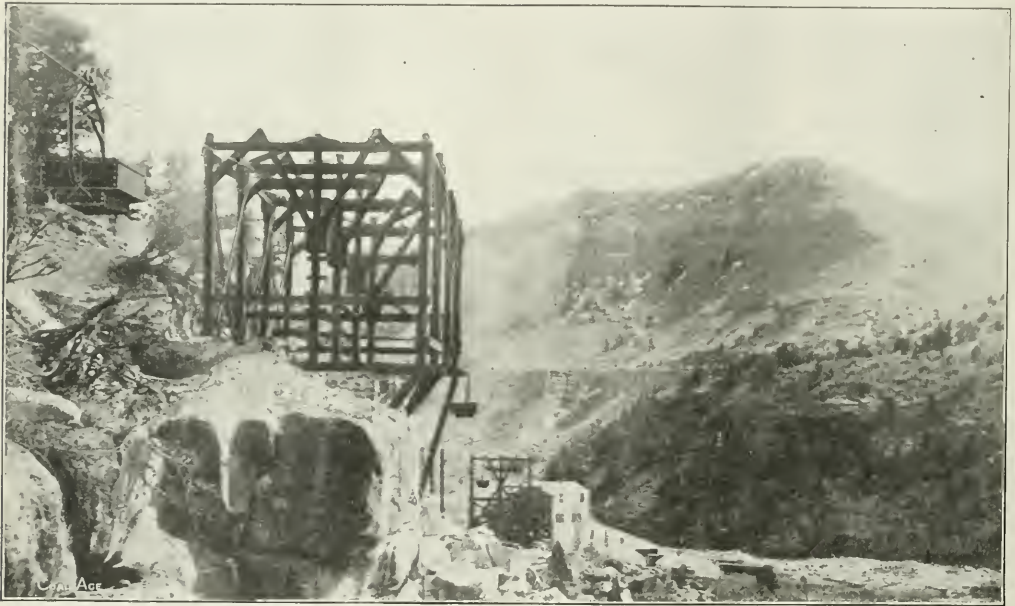
THE FOUR-SADDLE, OVERHANGING TOWER WHERE A DECIDED CHANGE IN GRADE IS MADE
