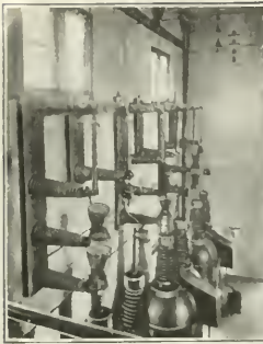
FIG. 10. CHOKE COILS IN TRANSFORMER HOUSE
