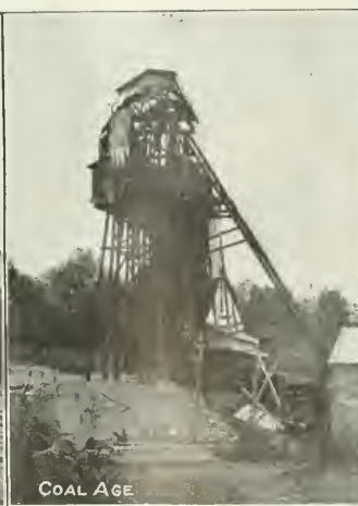
SHOWS DAMAGE DONE TO CLOVELLEY TIPPLE, VIGO COUNTY, IND., BY EXPLOSION ON NOV. 10
