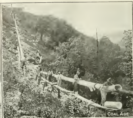
FIG. 13. PLACING THE COVERING ON ONE OF THE 10-IN. LINES
