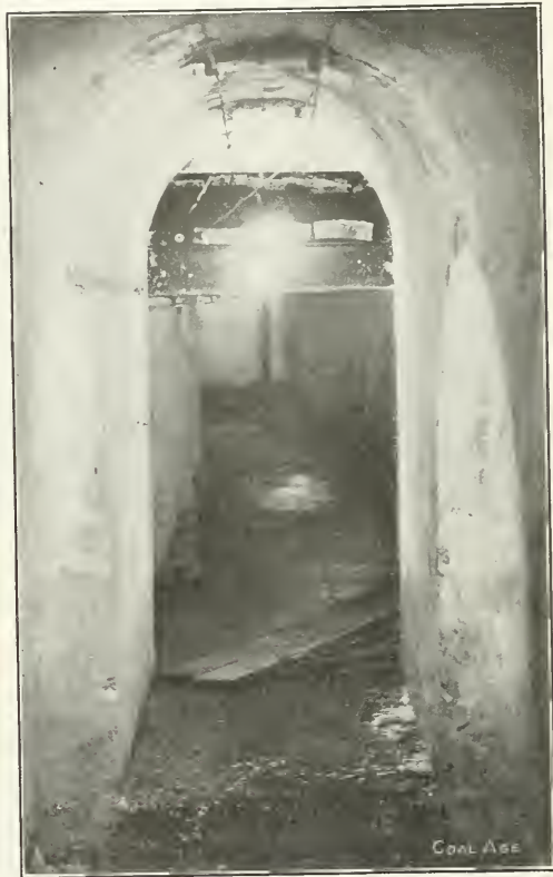
REINFORCED-CONCRETE RUN-A-ROUND AT THE No. 9 SHAFT BOTTOM
