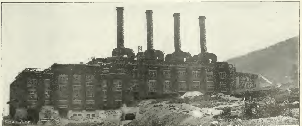
GENERAL VIEW OF THE ENTIRE BUILDING, SHOWING COAL TRESTLE AND SLUICE FOR CIRCULATING WATER
