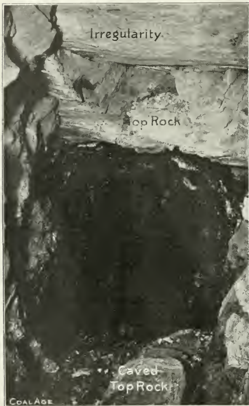
FIG. 7. INTERIOR OF TUNNEL SHOWING IRREGULAR MASSES OF FOREIGN MATERIAL IN ROOF
