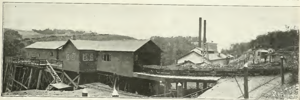
FIG. 1. TRIP ENTERING TIPPIE AND ABOUT TO BE DRAWN FORWARD BY THE TRIP PULLER
